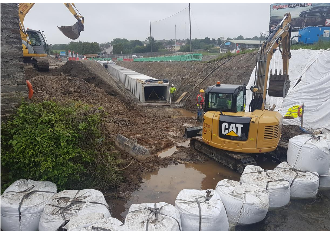
Example of a typical culvert being installed
