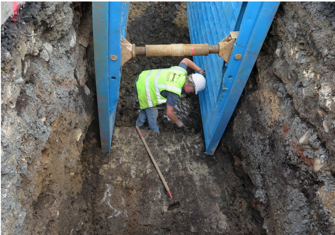
Figure 76 Investigating wall (C5-1A-15) in TT5-1A
