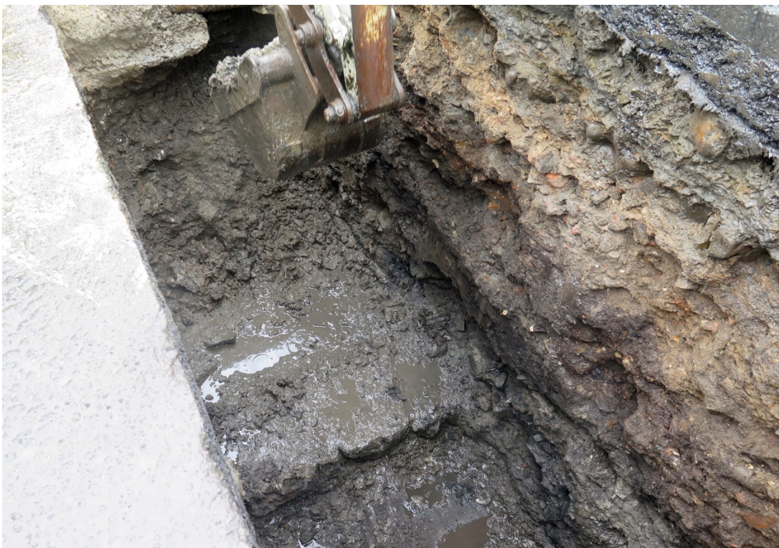
Figure 86 Quay wall revealed in the centre of TT5-2C
