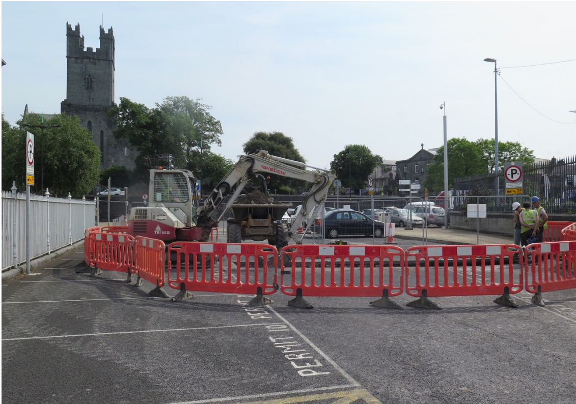
Figure 71 Location of TT5-1B, facing east towards St Mary's Cathedral
