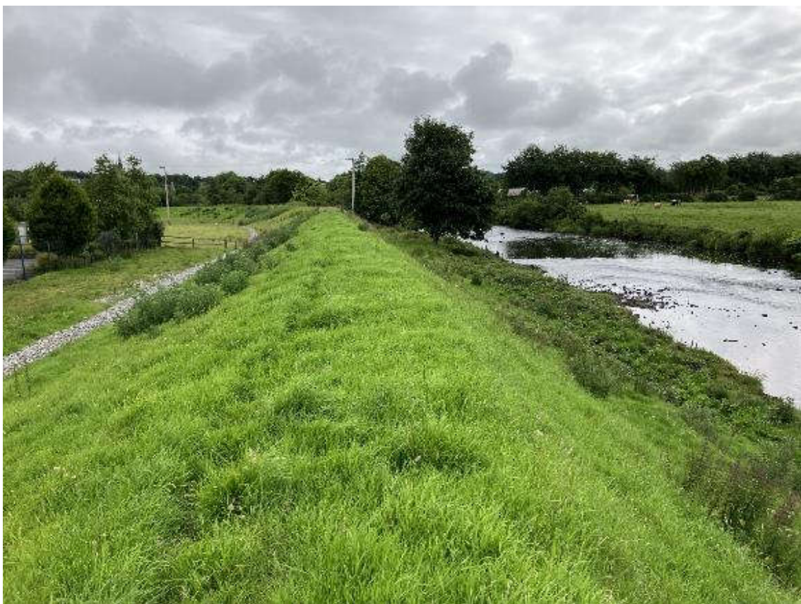
A recent photograph of the current condition of a section of the embankment near Finn Park, Ballybofey (June 2022)
