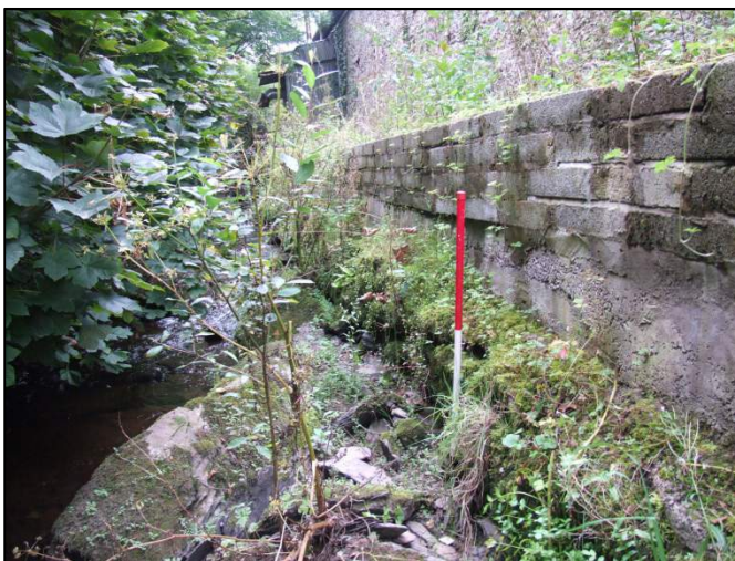
Plate 39: Southeast-facing view of modern block-work overlying the foundations of nineteenth-century river-walling on south side of the channel (1m scale).
