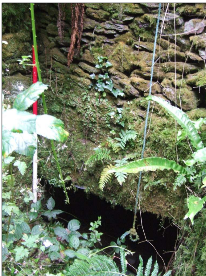
Plate 25: Southwest-facing view of masonry culvert accommodating flow the head-race to the tailrace, Feature F19, at Glen Mills/ Glen Distillery complex (1m scale).
