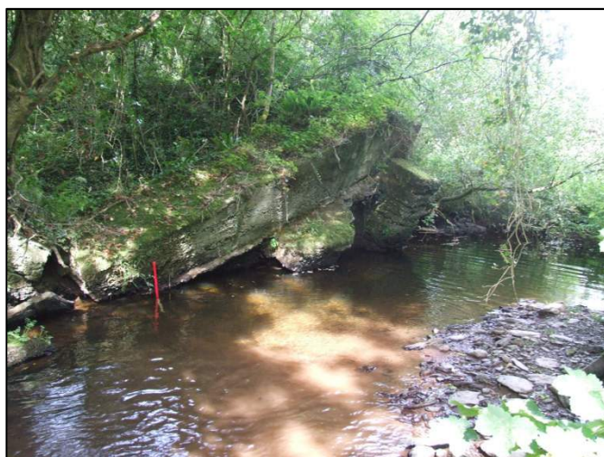
Plate 64: Northeast-facing view of the collapsed remains of a section of weir, Feature F26, located on the north side of the channel at NGR: 167061E, 75210N (1m scale).
