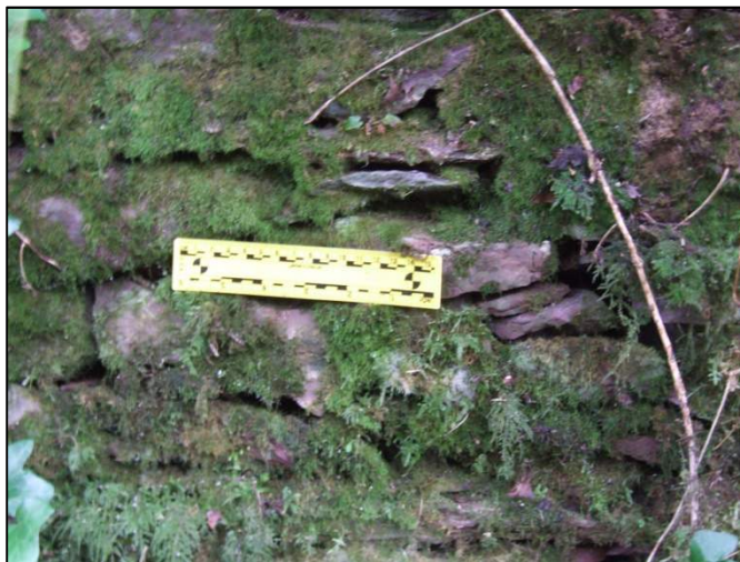
Plate 27: Detail shot showing lighter construction used for the upper part of the tailrace wall (150mm scale).
