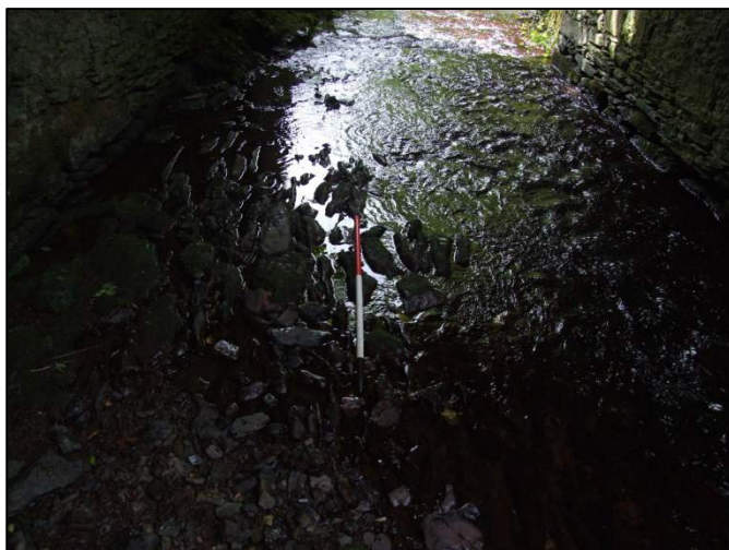
Plate 56: West-facing view of stone-lined apron covering the riverbed beneath bridge Feature F24 (1m scale).
