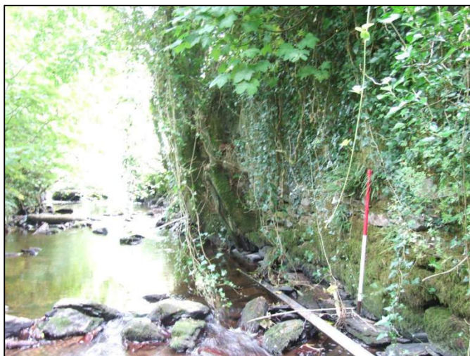
Plate 41: East-facing view of river channel where river-walling, Feature F22, survives to its original height (1m scale).
