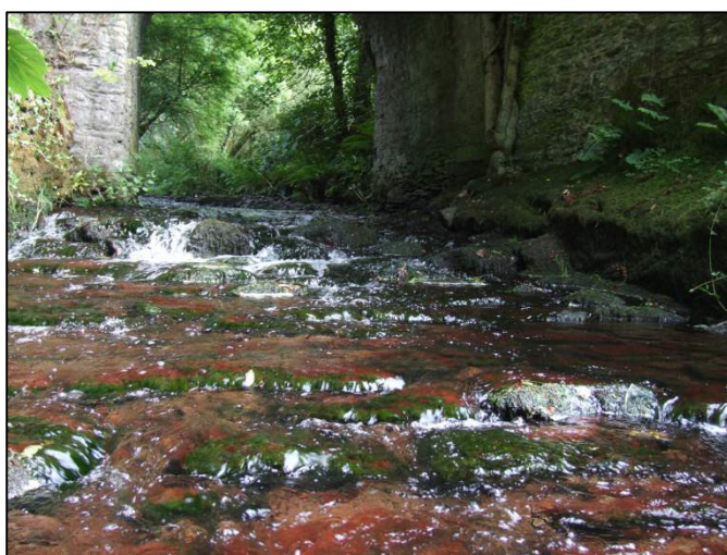
Plate 58: East-facing view of the stone-lined apron extending across the riverbed on the downstream side of the bridge, Feature F24.
