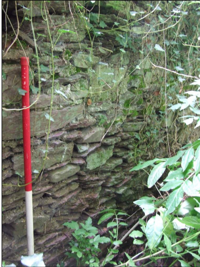
Plate 26: View of wall forming the north side of a tailrace, Feature F19, structure at the Glen Mills/ Glen Distillery complex (1m scale).
