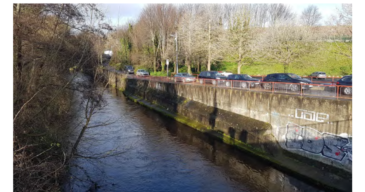
VIEW 2 ALONG EXISTING ACCESS ROAD
