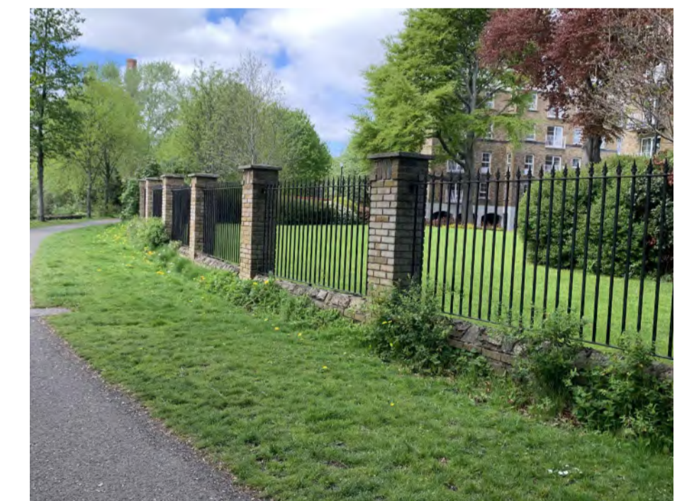
VIEW 2 ALONG SHANAGARRY APTS BOUNDARY WALL
