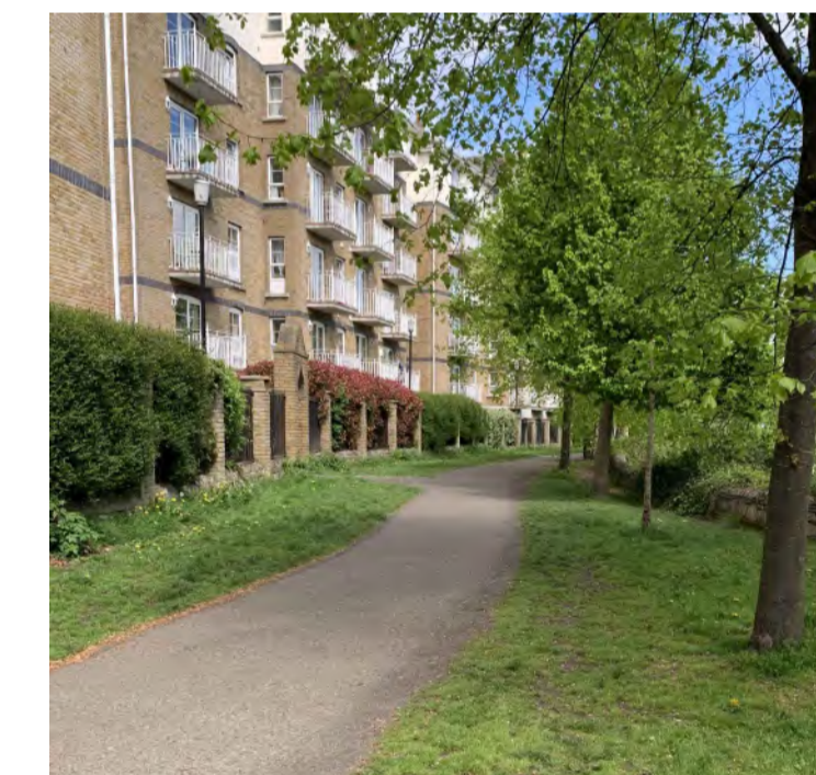
VIEW 1 ALONG SHANAGARRY APTS BOUNDARY WALL
