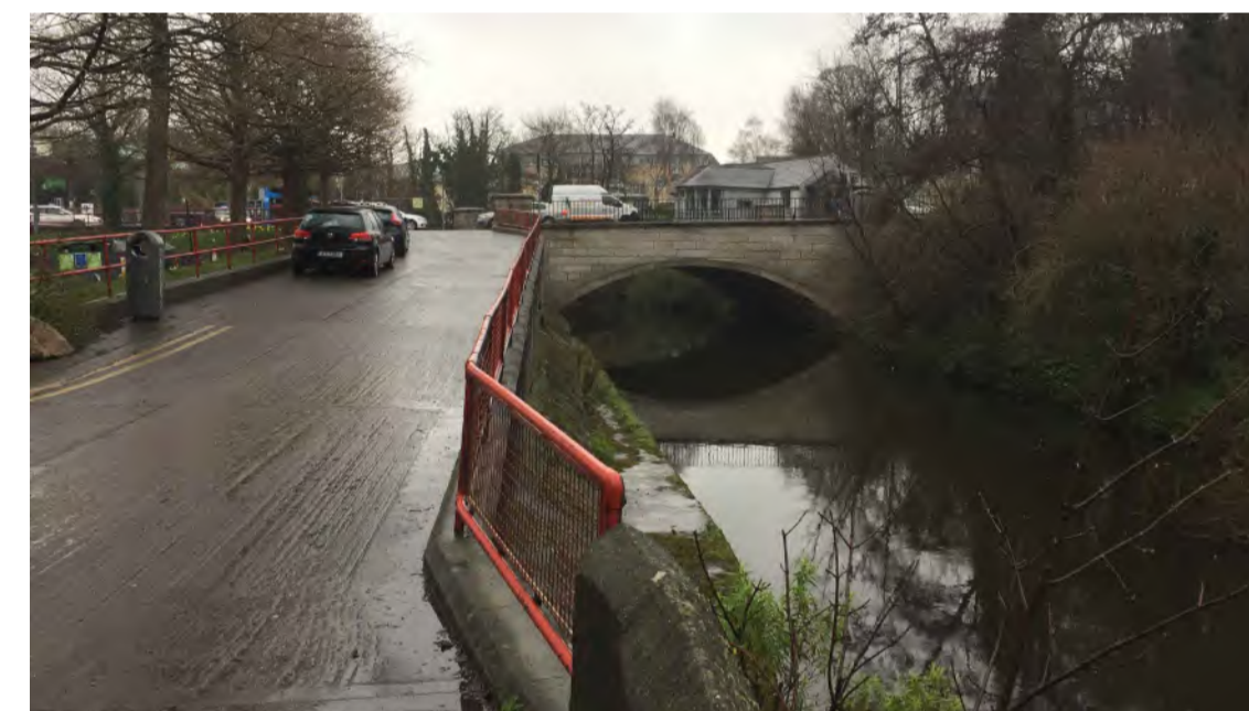
VIEW 1 ALONG EXISTING ACCESS ROAD
