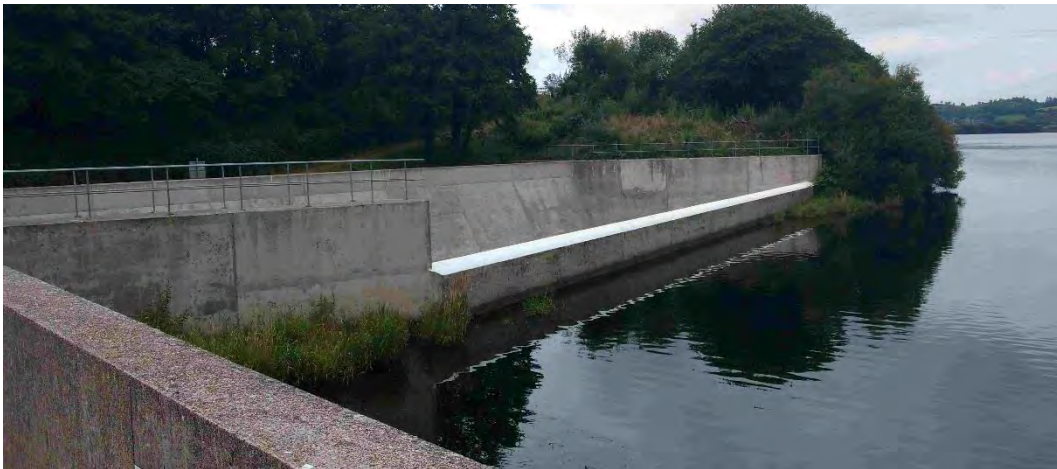
Figure 17: Carrigadrohid Auxiliary Spillway Ogee Weir
