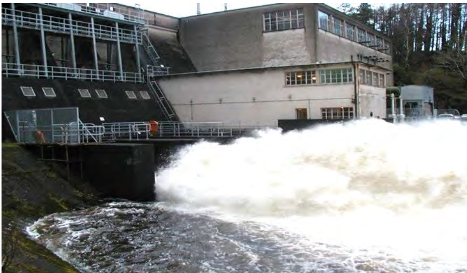
Figure 5: Carrigadrohid Hydropower Station (deep sluices in foreground)
