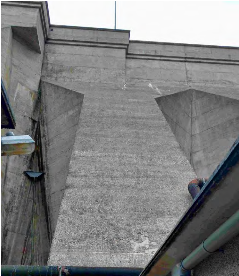
Figure 19: Downstream face of Inniscarra Dam, demonstrating complicated buttress geometry
