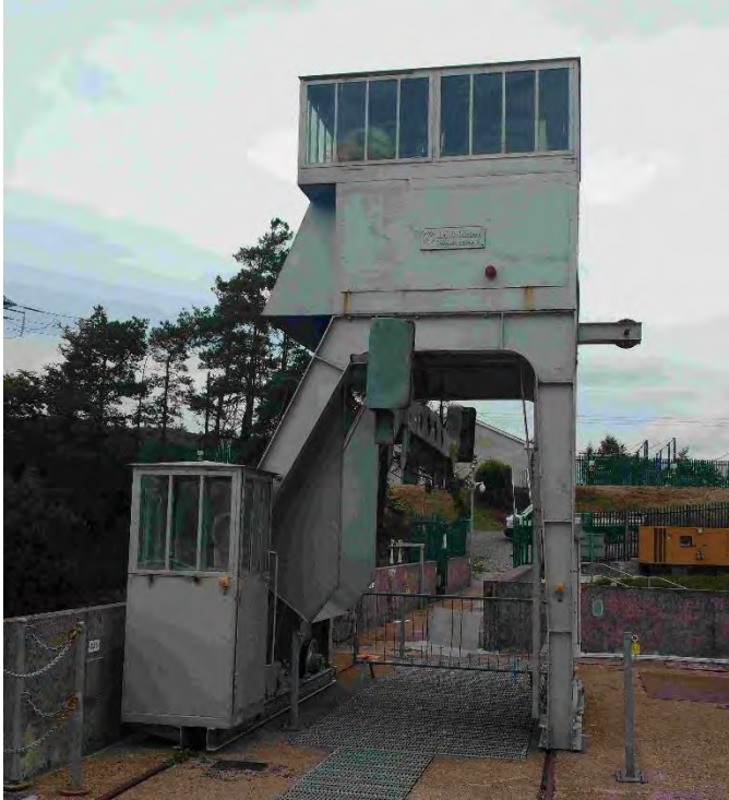
Figure 16: Carrigadrohid Dam Crest Gantry Crane
