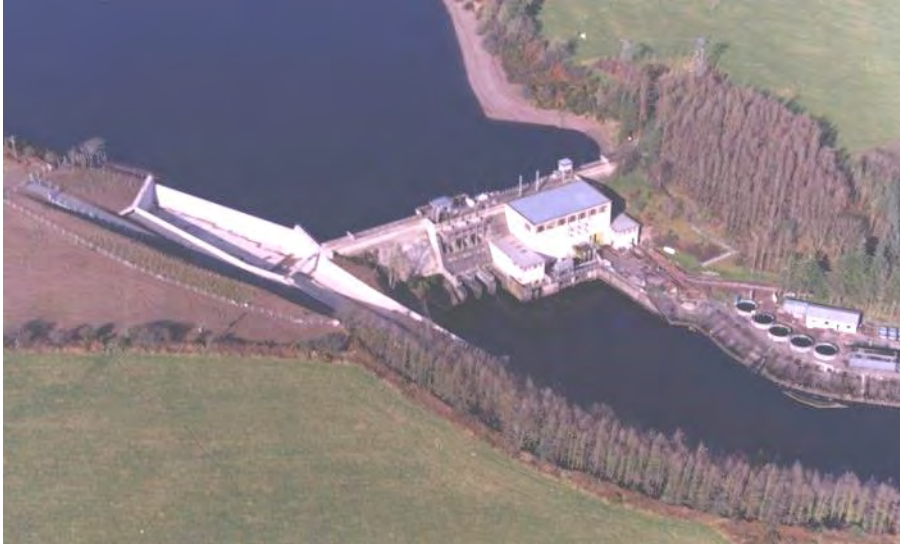
Figure 5: Carrigadrohid Hydropower Station (deep sluices in foreground)
