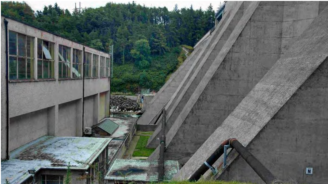
Figure 21: Downstream face of Inniscarra Dam at the intake blocks, demonstrating lack of working room between the dam and the turbine house
