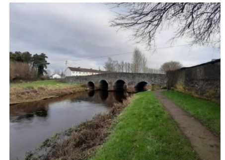
Figure 1 A view of Spa Street Bridge from the River Barrow Walk
