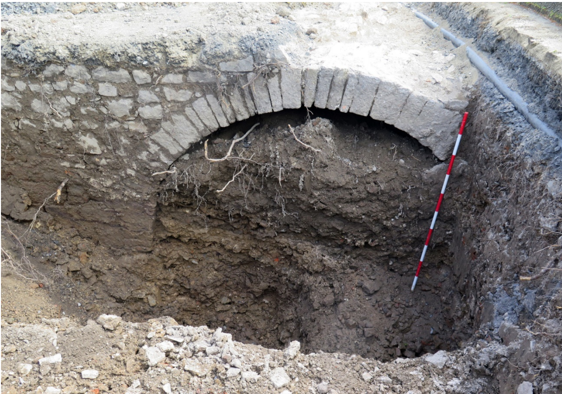
Figure 21 South-facing view of western arch C1-1-05
