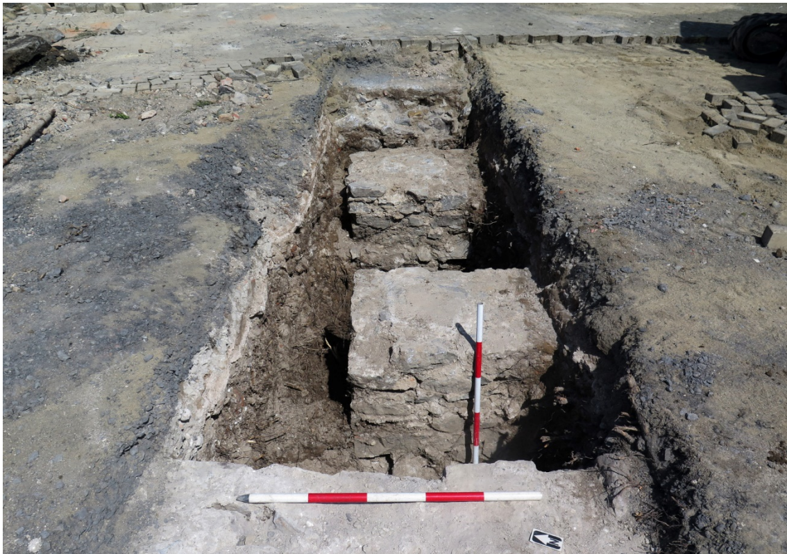
Figure 26 Looking east across TT1-3 showing foundation pads, C1-3-12 in foreground and C1-3-13 in background
