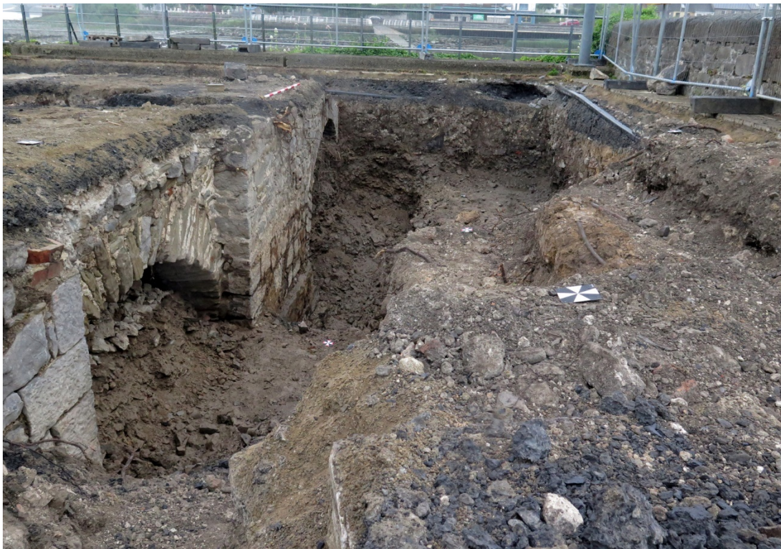
Figure 18 West-facing view of the north elevation of brewery building showing two arches, infilled in 1890s.
