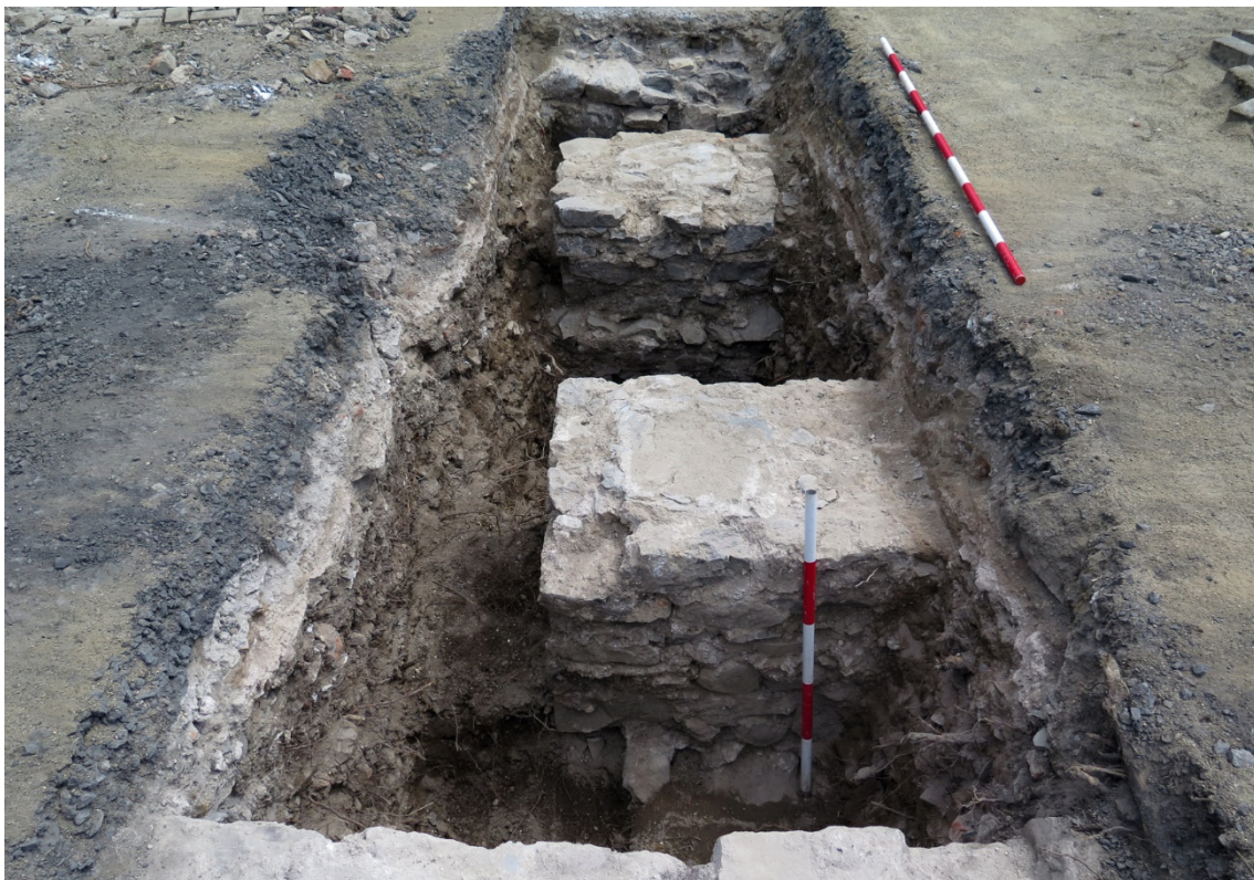
Figure 27 Elevation of C1-3-13 looking west
