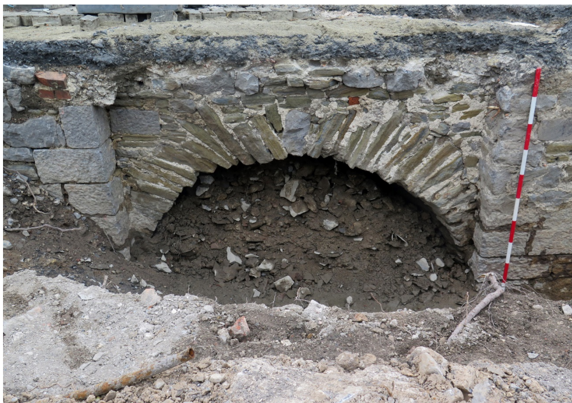
Figure 22 South-facing view of eastern arch C1-1-06
