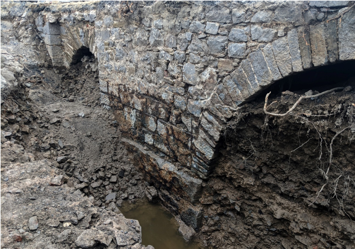
Figure 20 Southeast-facing view of arches showing foundation course.
