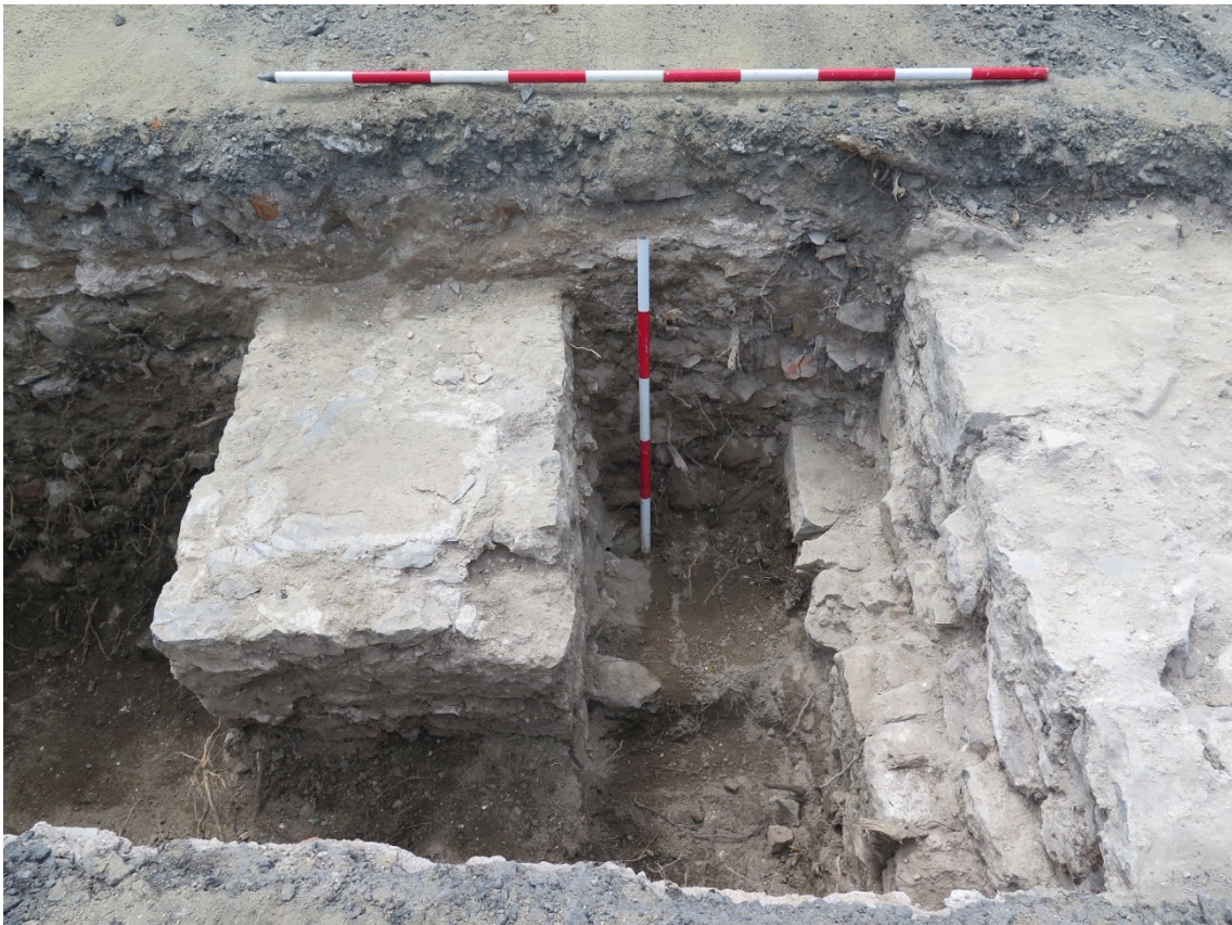
Figure 29 Facing south to abutment wall for western arch C1-3-15 and pad C1-3-12
