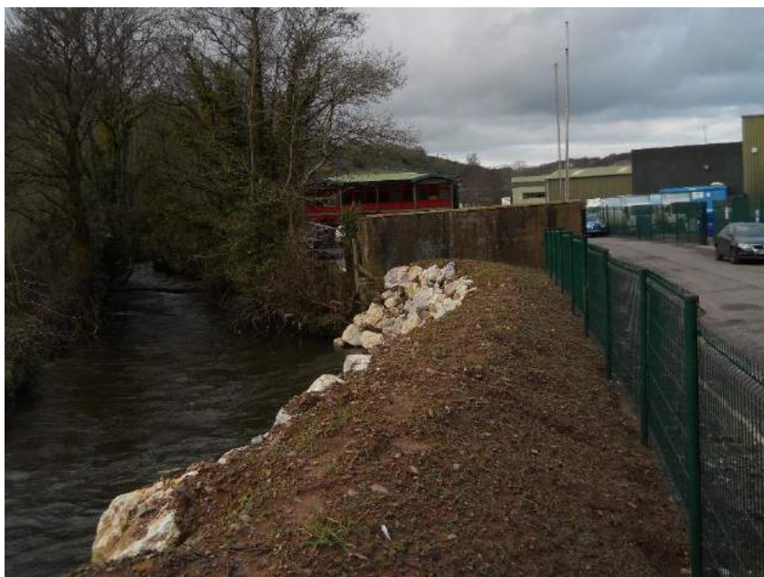
Figure 2-11 Defences constructed at Grandon Car Sales prior to the 2012 event
