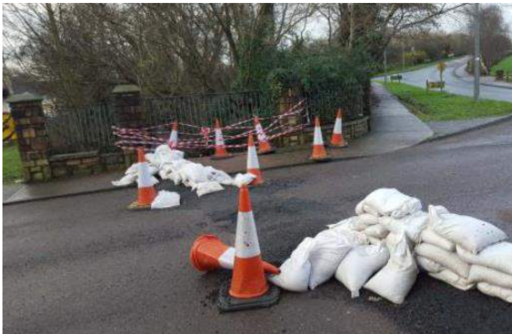
Figure 3-18: Emergency surface flow management measures at the entrance to Copper Valley Vue
