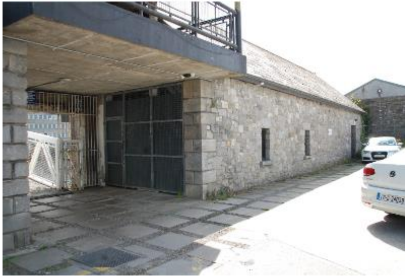
Plate 14-60. Interior of south wall in area of proposed ramp
