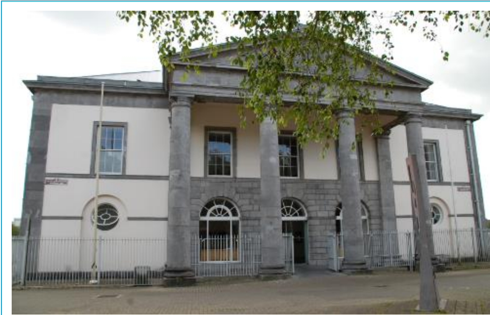
Plate 14-46. Front façade of County Court House, protected structure (RPS 012)
