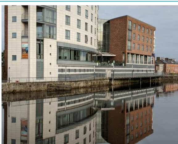
Plate 14-26. View looking north to Area 9 (left) which rises to access Area 8 (right), existing boardwalk. Southern extent of Area 7, Sir Harry's Mall in far right
