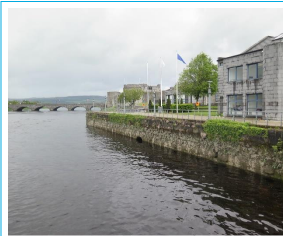
Plate 14-32. View of the Limerick City Council buildings, the location of the former city jail, facing north
