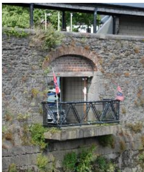
Plate 14-59. Opening in south wall
