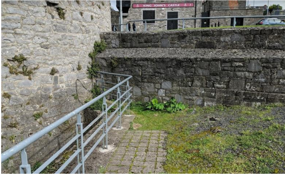
Plate 14-57. King John’s Castle, National Monument, RPS 004, showing existing railings, to be replaced with glass panels, with tie into the later wall to the right
