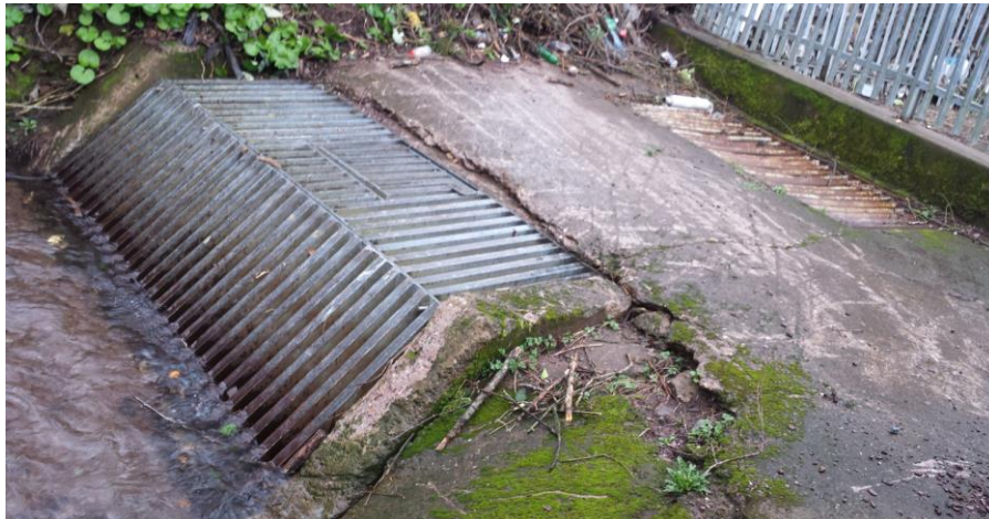
Figure 3: Existing trash screen at entrance to culvert in Lehenaghmore Industrial Estate
