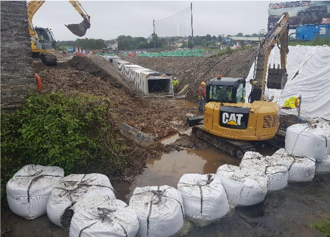
Example – Flow Diversion Culvert (under construction)
