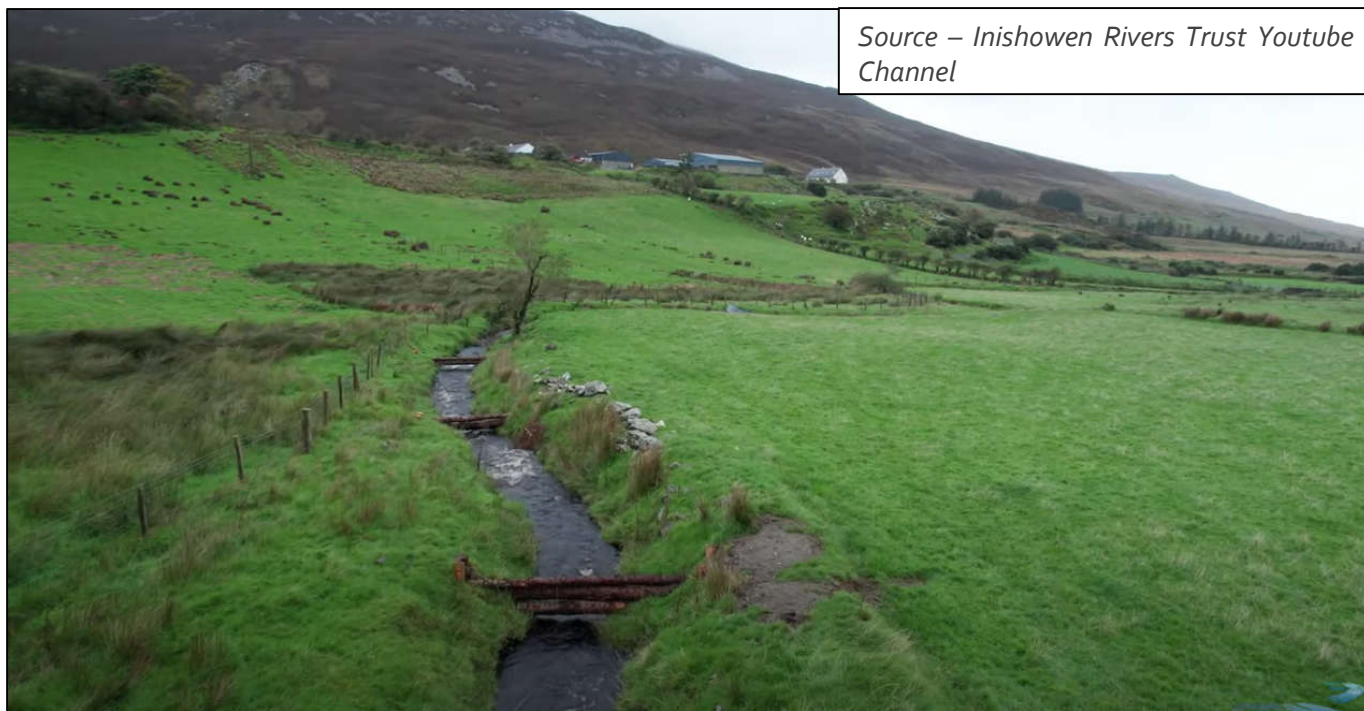
Leaky Dams in Inishowen (Example of Natural Water Flood Measures in the upper catchment) -
