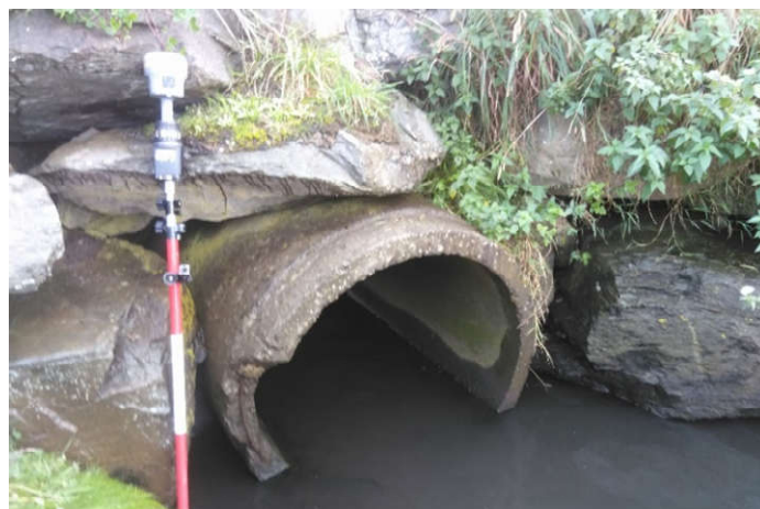
Culvert Condition Survey works, Buncrana
