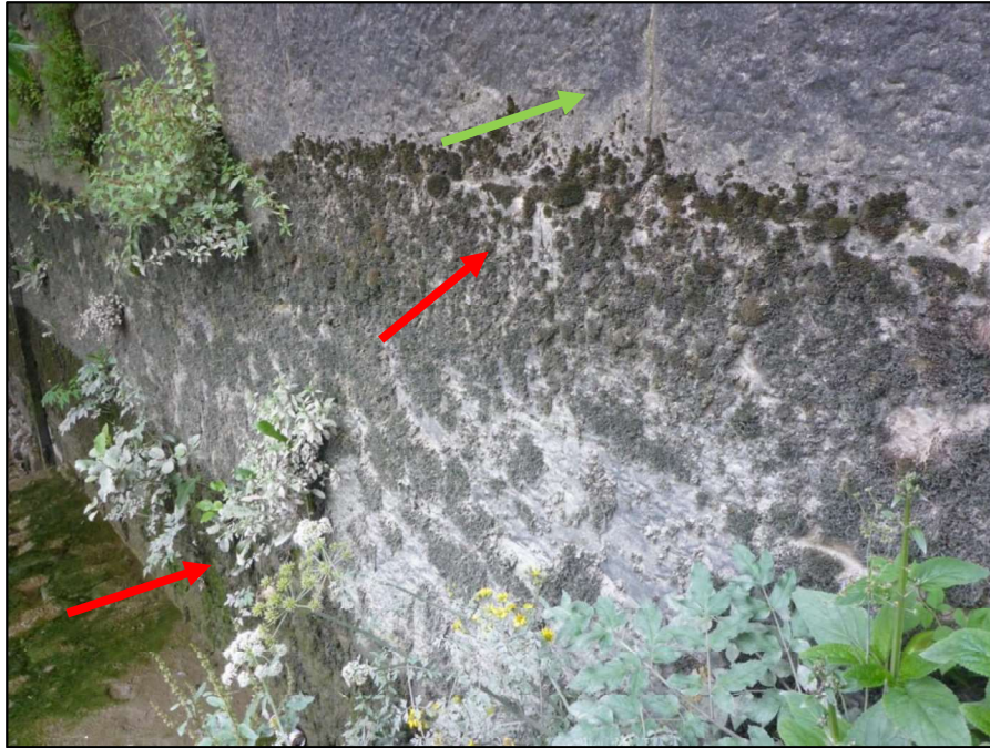
Photograph 4.2. Example of aquatic bryophyte zone on quay wall (red arrows) and non-aquatic bryophytes at the top of the high water line (green arrow)
