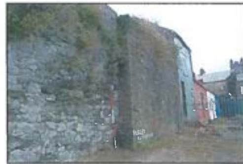
Plate 3.4. Verdant Place extra facing, from northeast
