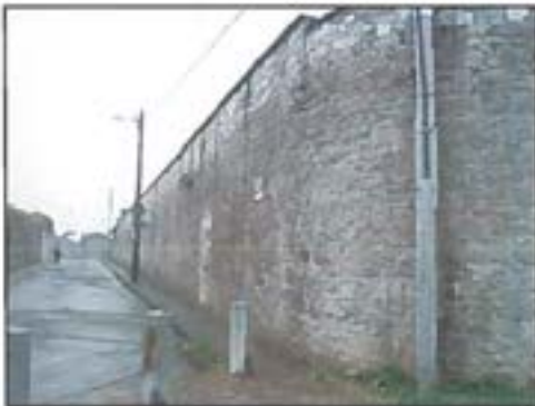
Plate 3.24. Location of Island Gate, from northwest
