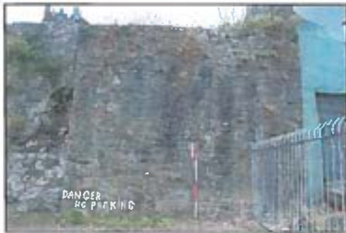
Plate 3.3. Verdant Place, extra facing added to City Wall, from west
