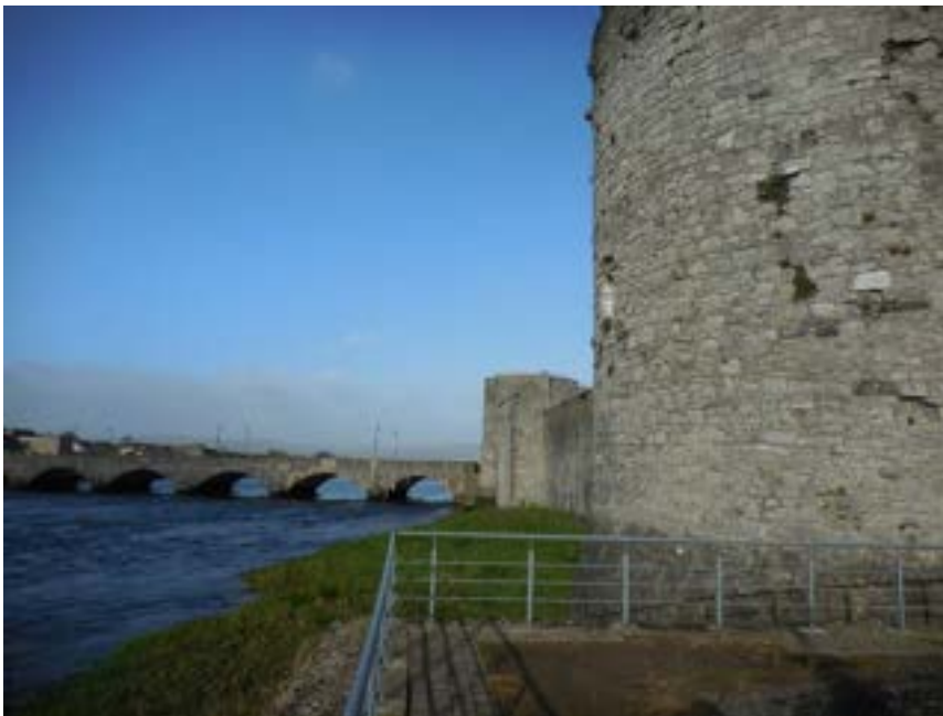
Plate 3 View along Curtain wall of King John's Castle
