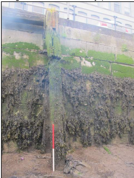
Plate 204: Example shot of timber fenders used along Father Matthew Quay/Morrison's Quay (1m scale).
