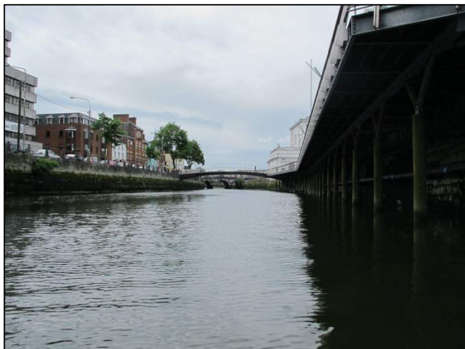
Plate 173: West-facing view of the south channel showing Sullivan's Quay on left of picture, Nano Nagle Bridge in distance.
