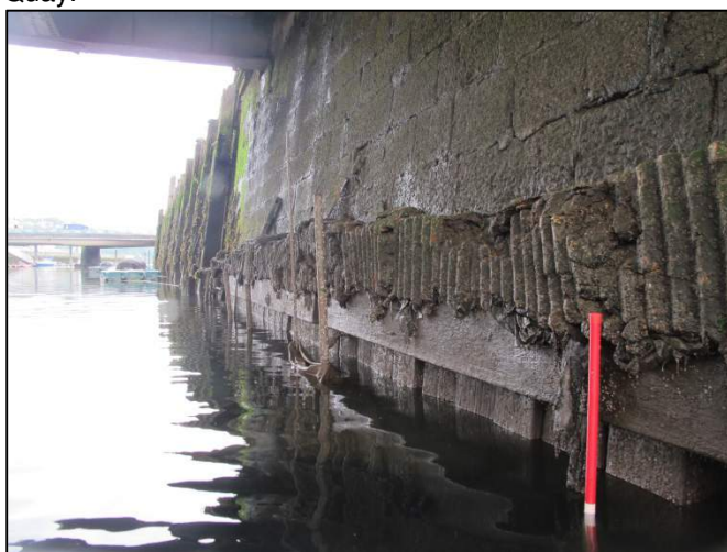
Plate 218: East-facing view along Albert Quay; shot taken beneath Clontarf Bridge. Note timber fenders running toward the timber wharf in distance (1m scale).
