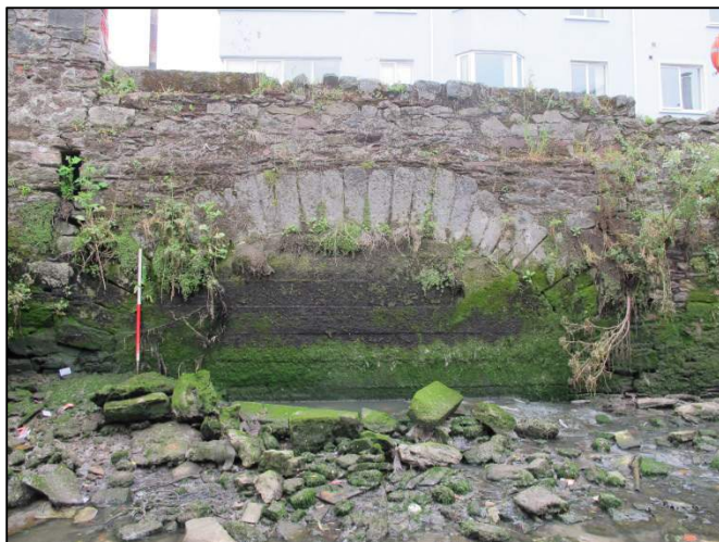
Plate 160: West-facing view of an arched-culvert located at the southern terminus of Crosse's Green Quay (150mm scale).
