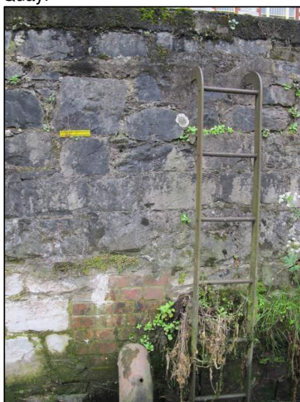
Plate 158: South-facing view showing the transition between the original quayside masonry and the later addition of a rubble-stone wall at Wandersford Quay (150mm scale).
