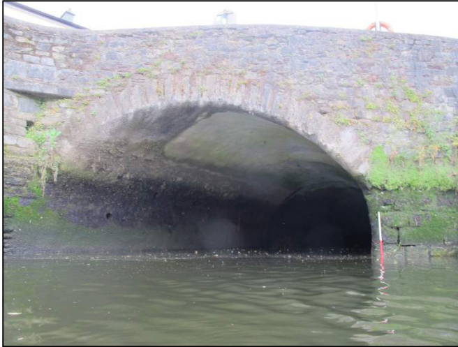
Plate 166: West-facing view of an arched-culvert located at the upstream end of French's Quay (1m scale).
