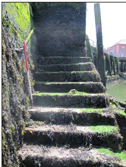
Plate 193: West-facing view of a flight of river-access steps located at the upstream end of Union Quay (1m scale).
