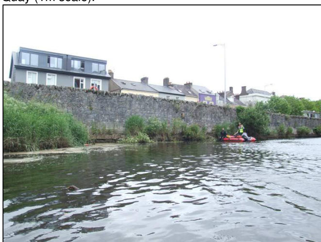
Plate 153: Northeast-facing view along an upstream section of Lancaster Quay.
