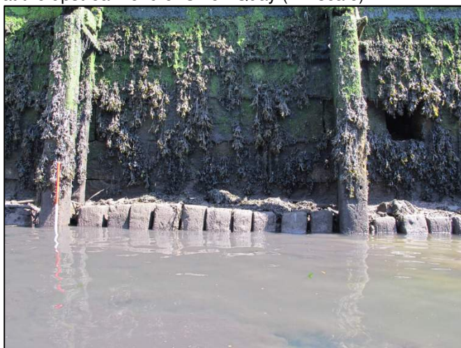
Plate 194: South-facing view of timber piles used to underpin the quay wall (1m scale).
