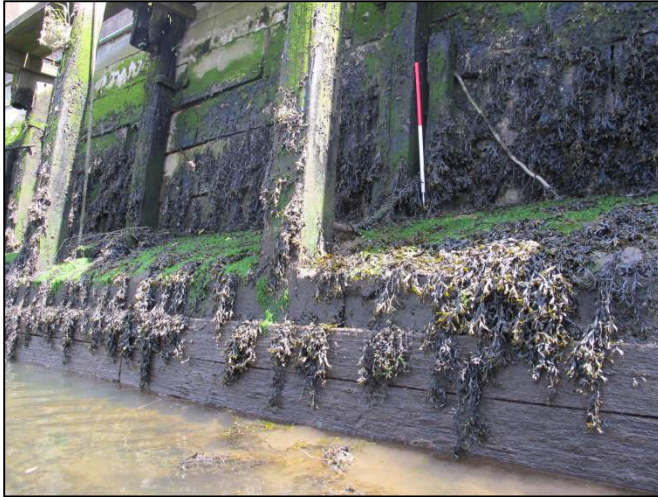
Plate 190: Southeast-facing view of timber shuttering and concrete used to underpin Union Quay at the location of timber wharf (1m scale).
