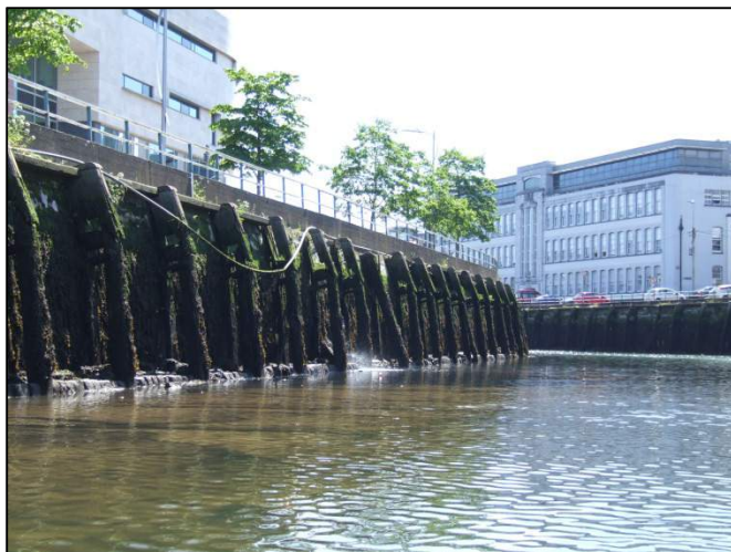
Plate 196: Southwest-facing view of timber fenders running along Union Quay.
