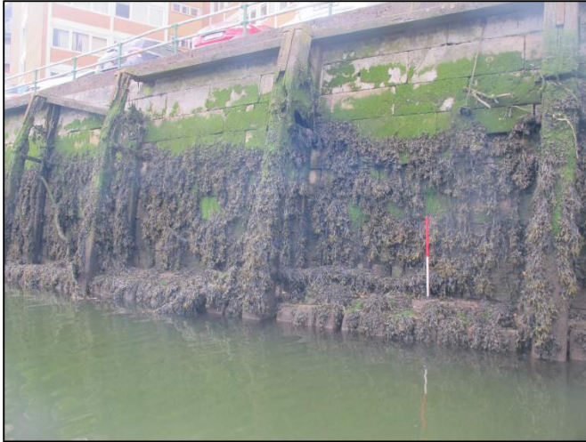
Plate 202: Example shot of timber piles and concrete used to underpin section of Father Matthew Quay/Morrison's Quay (1m scale).
