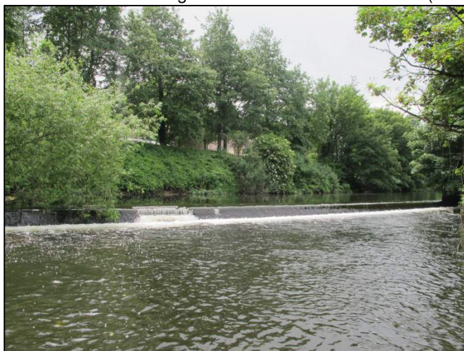
Plate 225: West-facing view of Weir F051 (Gill Abbey Weir).
