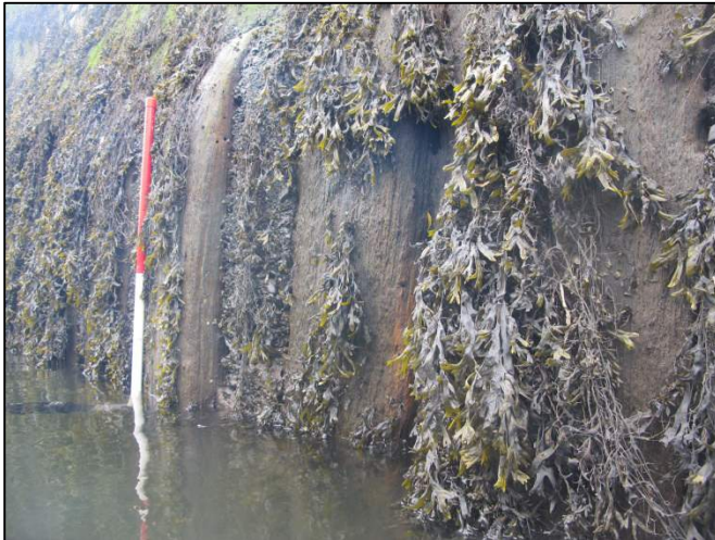
Plate 203: Example shot of timber piles set flush to the quay wall along Father Matthew Quay (1m scale).
