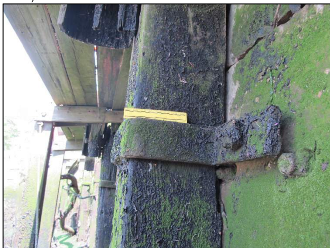
Plate 188: Detail shot showing iron strap-fastenings used to secure wharf timber to the quayside (150mm scale).
