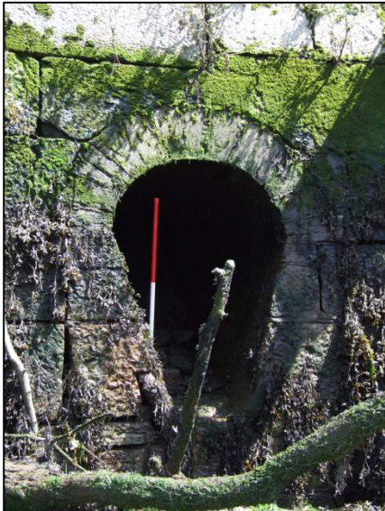
Plate 191: South-facing view of keyhole-shaped arched-culvert located along the upstream side of Union Quay (1m scale).
