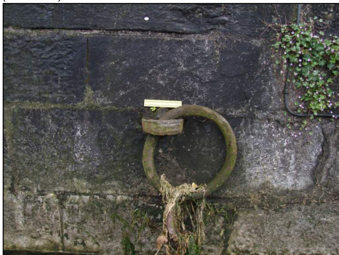
Plate 179: Example of wrought iron mooring-rings located along Georges Quay (150mm scale).
