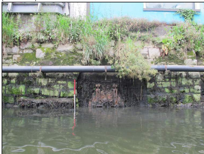
Plate 176: North-facing view of arched culvert located at the terminus of an unnamed quay on the South Mall, F039 (1m scale).
