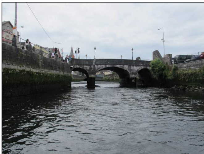
Plate 172: West-facing view along Sullivan's Quay on the upstream side of Nano Nagle Bridge, South Gate bridge in distance.
