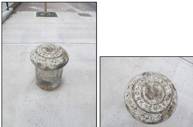
Plate 214: Example shot of one of the mooring bollards located at Albert Quay (1m scale).
