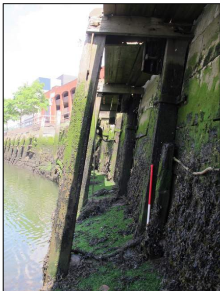
Plate 187: East-facing view of a section of timber wharf located at Union Quay, immediately downstream of Trinity Footbridge (1m scale).
