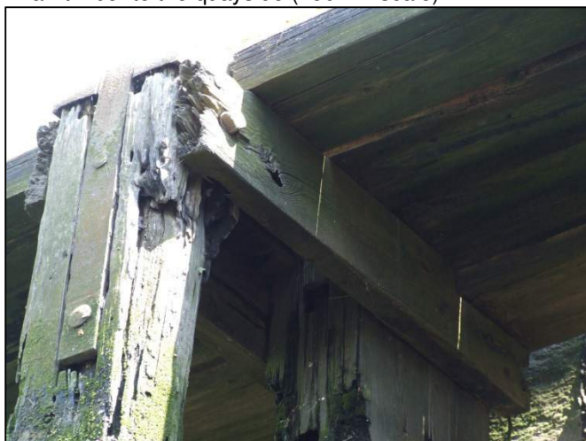
Plate 189: Detail shot showing the timber assemblage that supports the wharf's timber deck.
