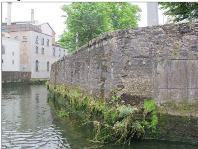
Plate 155: South-facing view showing the downstream terminus of Wandersford Quay, where it con-joints with the northern end of Crosse's Green Quay (1m scale).
