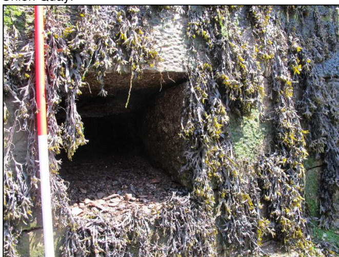
Plate 197: Example shot of drain features located along Union Quay (1m scale).
