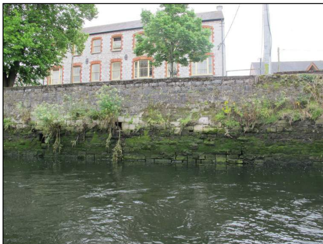
Plate 157: South-facing view showing the fabric of Wandersford Quay.
