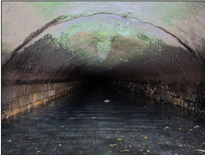
Plate 167: Internal view of the culvert structure located at the upstream end of French's Quay.
