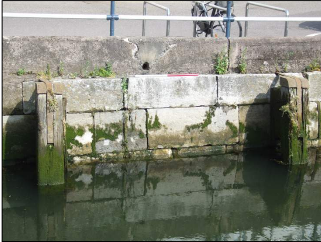
Plate 205: Example shot showing the top components of the timber fenders used along Father Matthew Quay/Morrison's Quay (1m scale).
