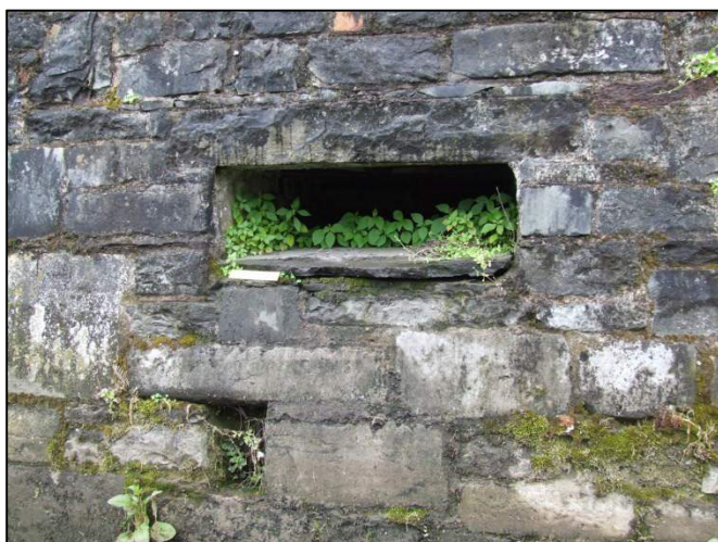
Plate 164: Detail shot of drain feature located along French's Quay (150mm scale).
