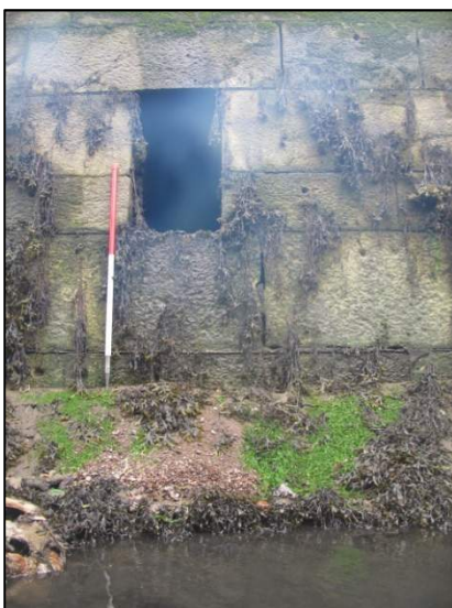
Plate 207: Example shot showing one of the rectangular drain features located along Father Matthew Quay/Morrison's Quay (1m scale).
