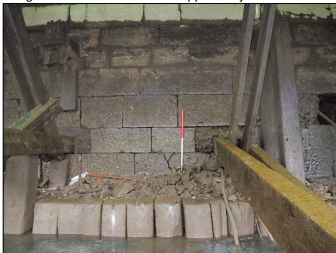
Plate 213: South-facing view showing fabric of Albert Quay beneath an adjoin timber wharf (1m scale).
