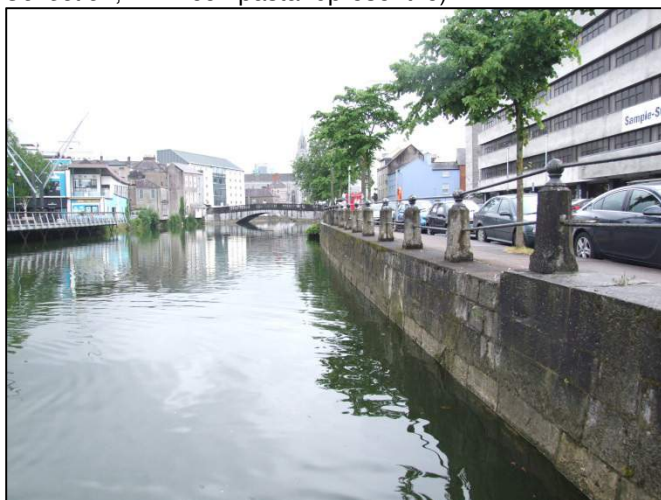
Plate 171: East-facing view along Sullivan's Quay on the downstream side of Nano Nagle Bridge.
