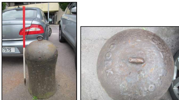
Plate 211: Example shot of one of the mooring bollards located at Lapp's Quay (1m scale).
