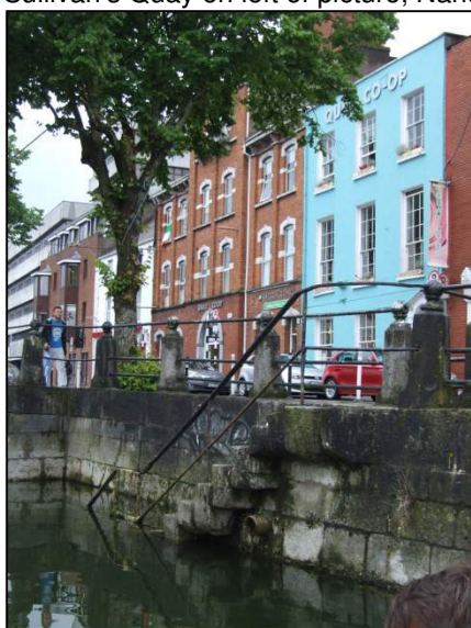
Plate 174: Flight of river-access steps built into Sullivan's Quay.
