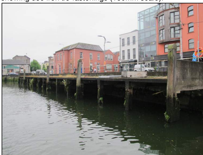
Plate 183: East-facing view of composite timber/concrete wharf located along the downstream side of George's Quay.
