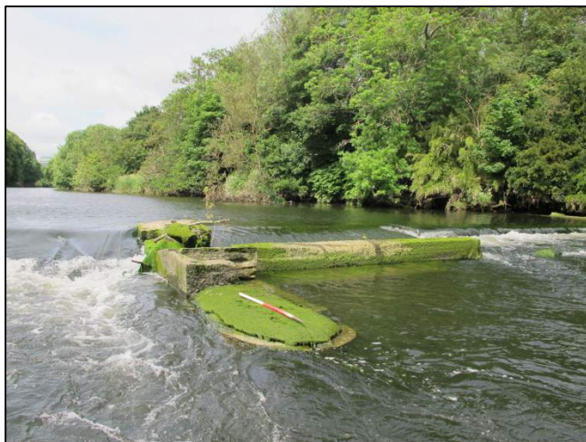
Plate 223: West-facing view of remains of fish-pass at Weir F049 (1m scale).
