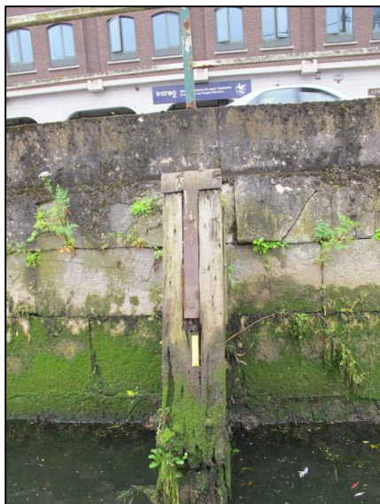
Plate 181: South-facing view of timber fender from George's Quay showing iron fastening at the top of timber (150mm scale).
