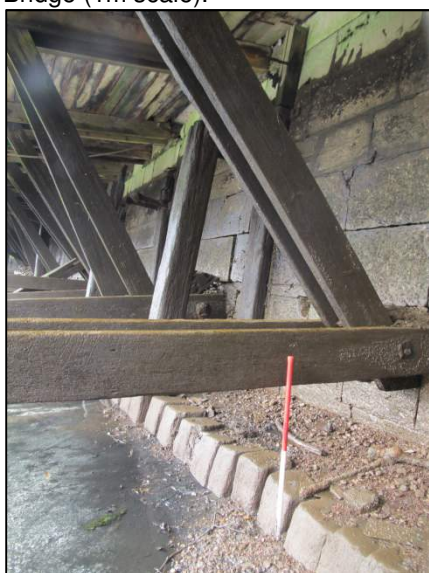
Plate 216: East-facing view of the timber wharfs sub-structure (1m scale).
