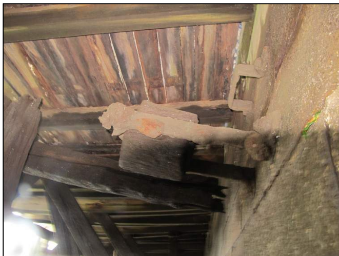
Plate 217: View along the underside of the timber wharf at Albert Quay.
