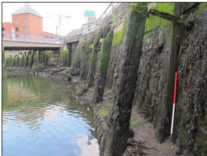
Plate 184: East-facing view of timber fenders located at the downstream terminus of George's Quay (1m scale).
