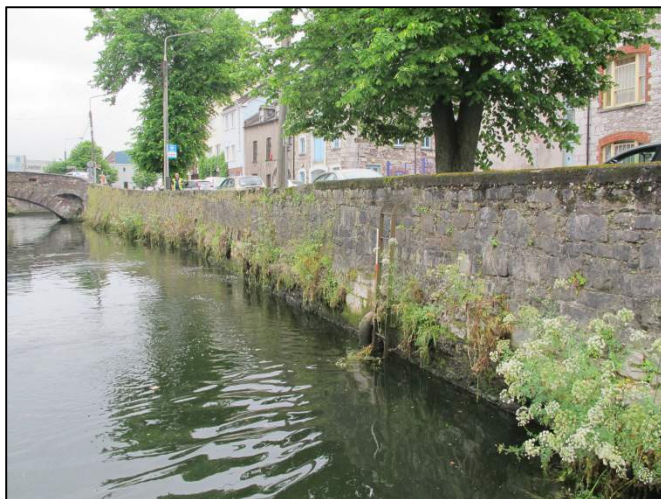
Plate 154: East-facing view along section of the original quayside forming Wandersford Quay (1m scale); Clarke's Bridge in background.
