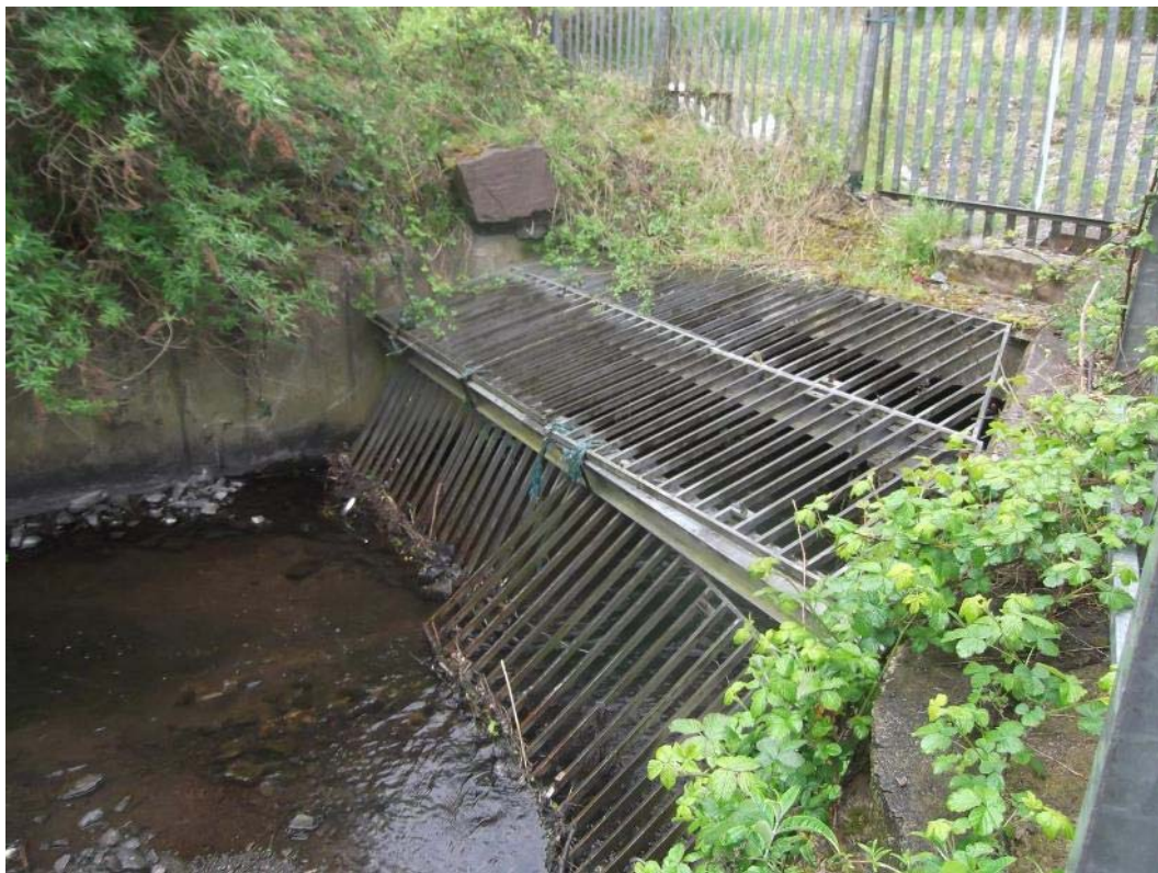
Figure 29 Existing trash screen on the Glen River at Spring Lane
