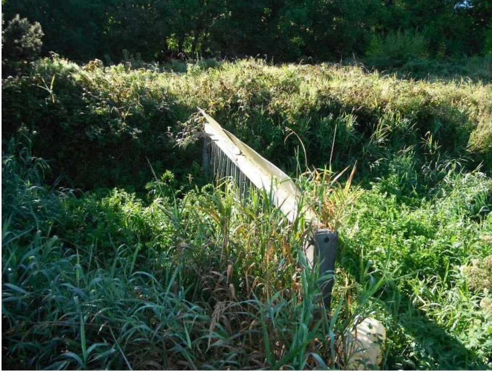
Figure 28 Existing Coarse Screen on Bride upstream of Glenamought confluence
