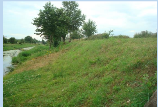
Existing Embankments in Limerick City
