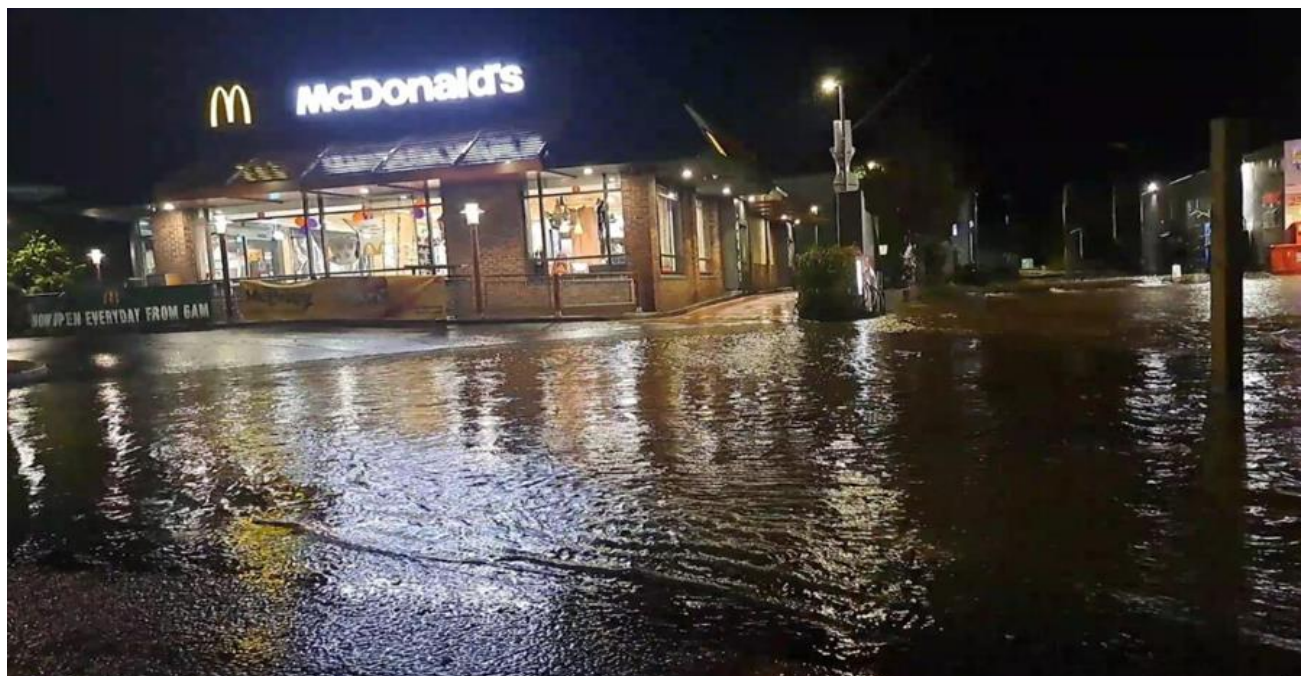
Flood at McDonalds on N3, October 2022
