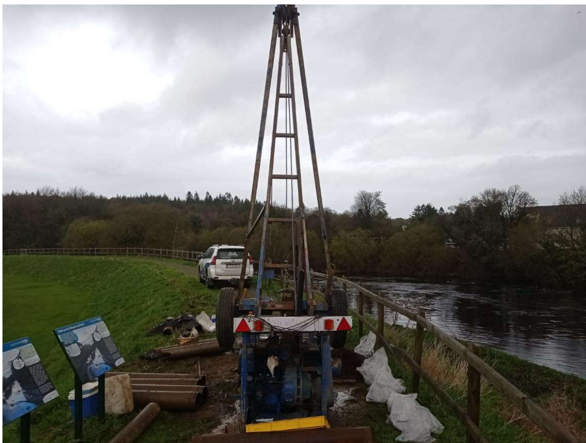
Cable Percussion Drilling along Ballybofey embankment, November 2022.
