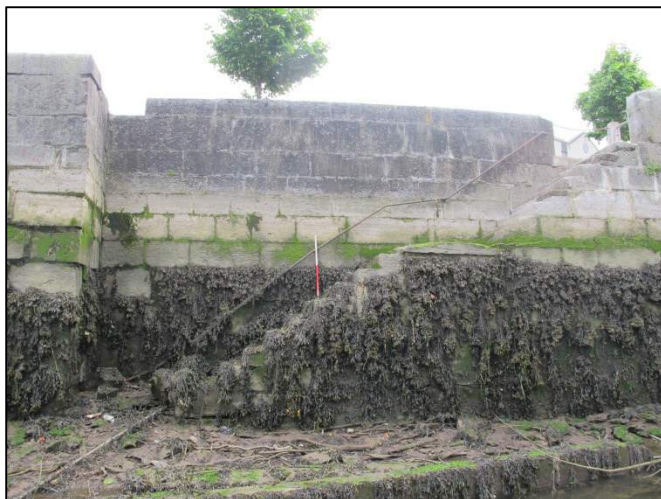
Plate 103: South-facing view of downstream flight of river access steps at Kyril's Quay (1m scale).
