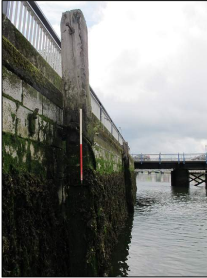
Plate 145: West-facing view of timber fenders attached to Anderson's Quay on the downstream side of Brian Boru Bridge (1m scale).
