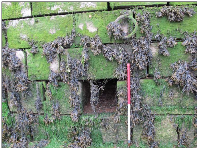
Plate 97: North-facing detail view of a mooring ring and drain feature at Pope's Quay (1m scale).
