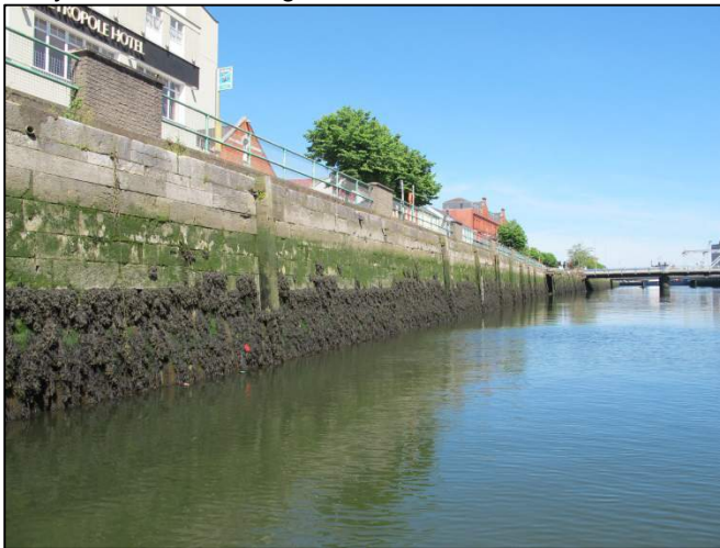
Plate 125: East-facing view of historic section of St. Patrick's Quay, Brian Boru Bridge in the distance.
