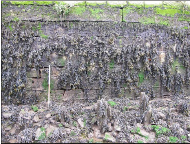
Plate 89: Detail view of original timber piles and shuttering used to underpin the quay's foundations (1m scale).
