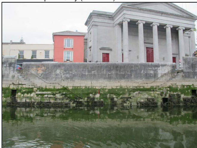
Plate 98: North-facing view of two opposing river access steps located a short distance upstream from the eastern terminus of Pope's Quay (1m scale).
