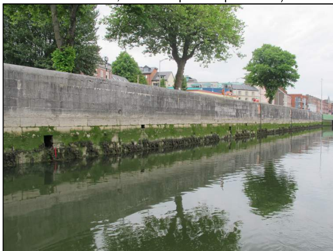
Plate 107: Northeast-facing view of Camden Quay on the upstream of Christy Ring Bridge (1m scale).
