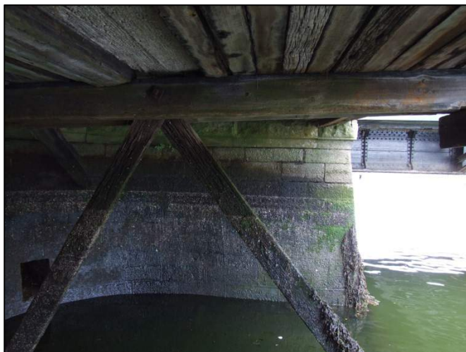
Plate 148: East-facing view of underside of timber wharf showing use of cross-braced timbers.
