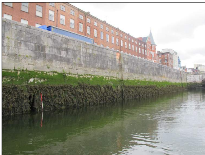
Plate 109: Northeast-facing view of Camden Quay, upstream of St. Patrick's Bridge (1m scale).
