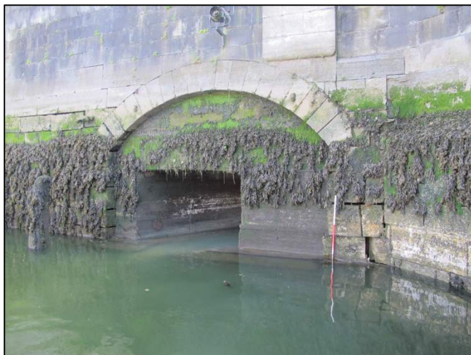
Plate 136: South-facing view of large arched-culvert located immediately downstream of St. Patricks Bridge (1m scale).
