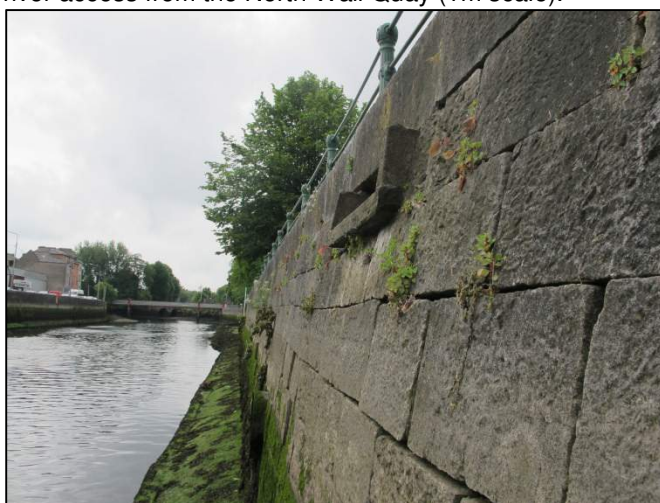
Plate 84: Drain feature located beneath the coping stones to provide drainage from the adjacent roadway.
