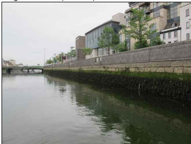
Plate 117: Southeast-facing view of Coal Quay/ Lavitt's Quay with Christy Ring Bridge in distance (1m scale).
