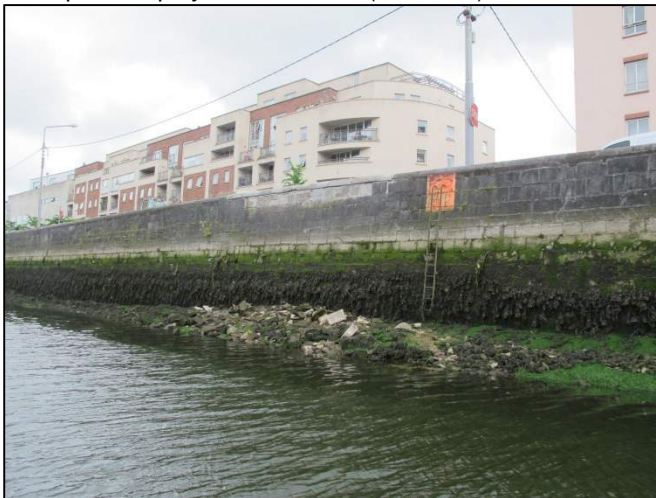
Plate 90: Southeast-facing showing location of modern quayside repair and collapsed masonry at the base of the quay wall.
