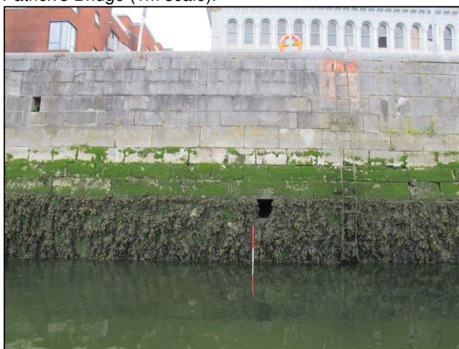
Plate 110: North-facing view of Camden Quay showing drain features and modern access ladder (1m scale).
