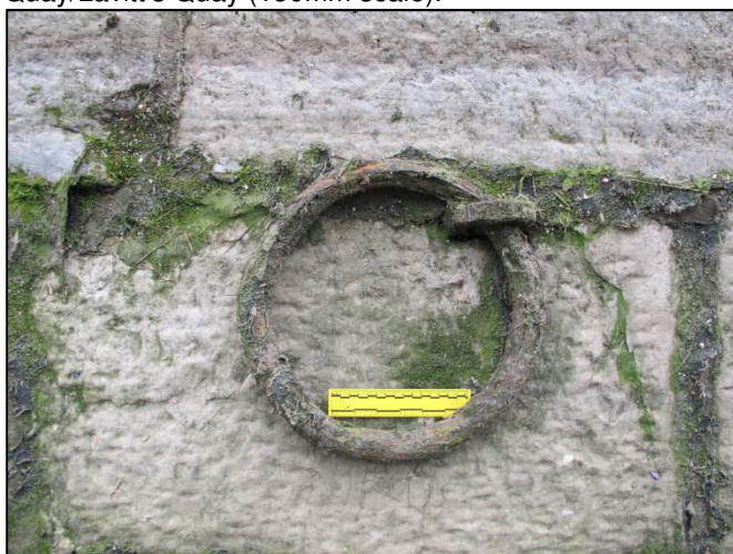
Plate 120: Example shot of mooring-rings present along Coal Quay/Lavitt's Quay (150mm scale).
