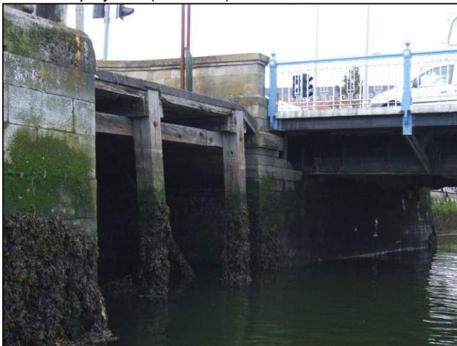
Plate 147: Southeast-facing view of a short section of timber wharf located on the downstream side of Brian Boru Bridge.
