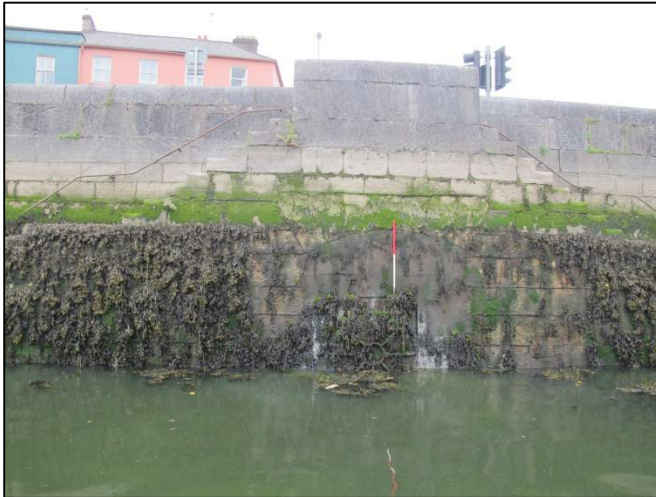
Plate 122: South-facing view showing arched culvert located between the two flights of steps (1m scale).
