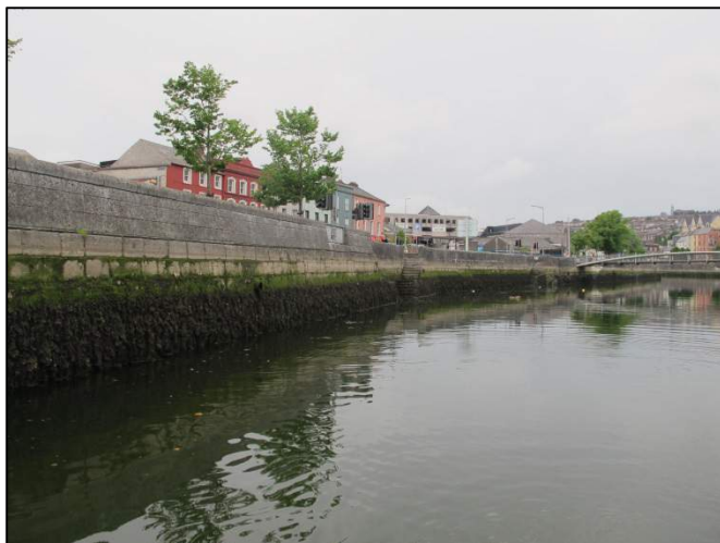
Plate 115: Southwest-facing view of Coal Quay with Shandon Bridge in distance.
