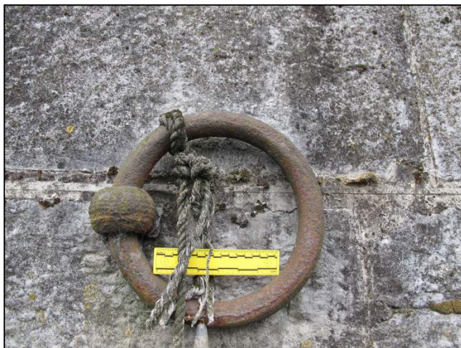
Plate 112: Example shot of drain mooring-rings located along Camden Quay (150mm scale).
