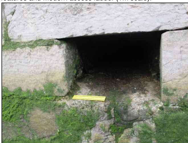
Plate 111: Example shot of drain features located along the High Water Mark at Camden Quay (150mm scale).
