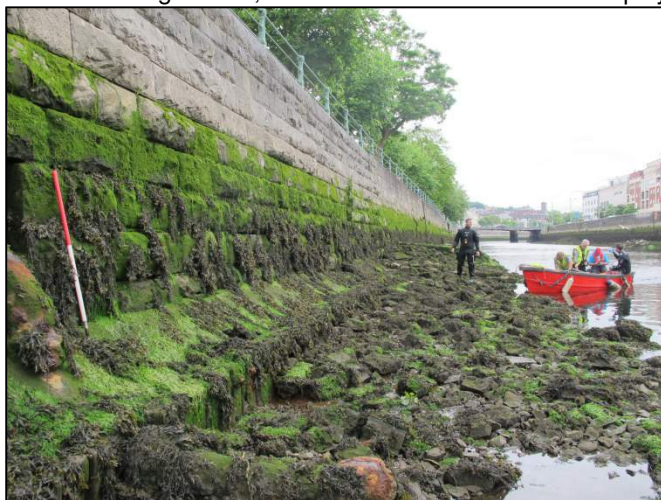
Plate 78: East-facing view along Wise's Quay (1m scale).
