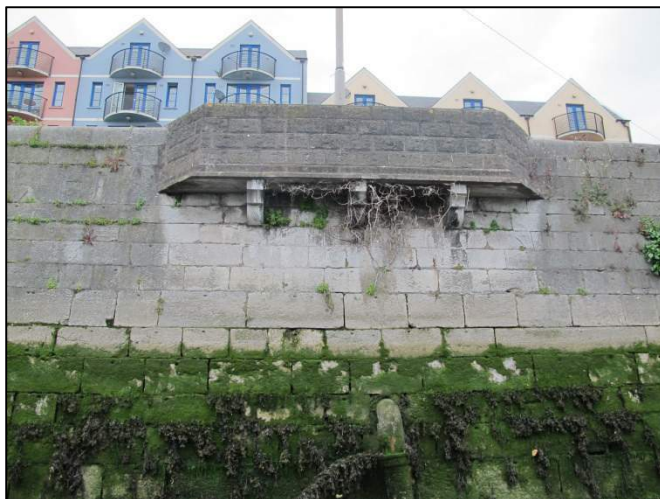
Plate 94: North-facing shot of viewing area built into the quay wall.
