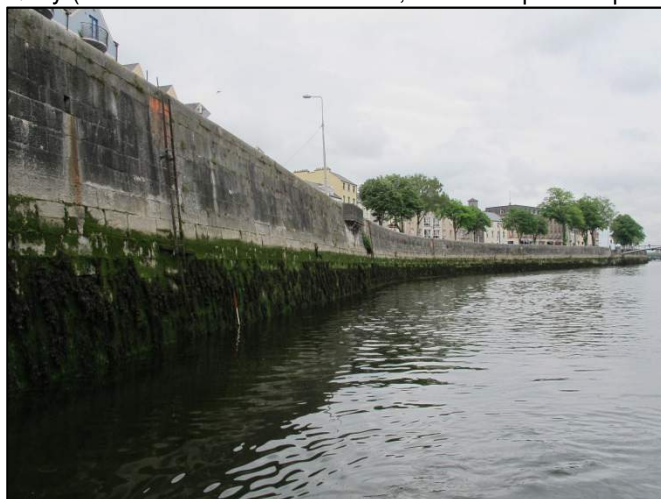
Plate 92: Northeast-facing view along the quay wall forming Farren's Quay leading onto Pope's Quay (1m scale).
