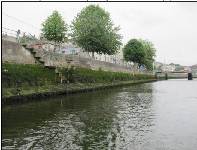
Plate 81: East-facing view along North Wall Quay (1m scale).
