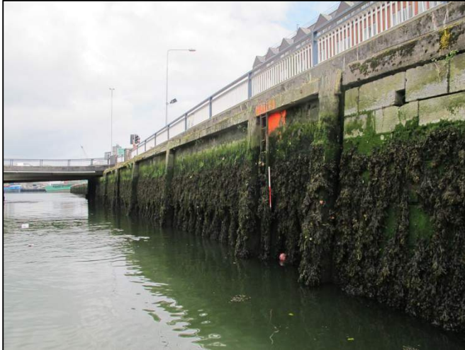
Plate 146: East-facing view of Anderson's Quay at a point where the historic masonry terminates and is replaced by a modern concrete quayside (1m scale).
