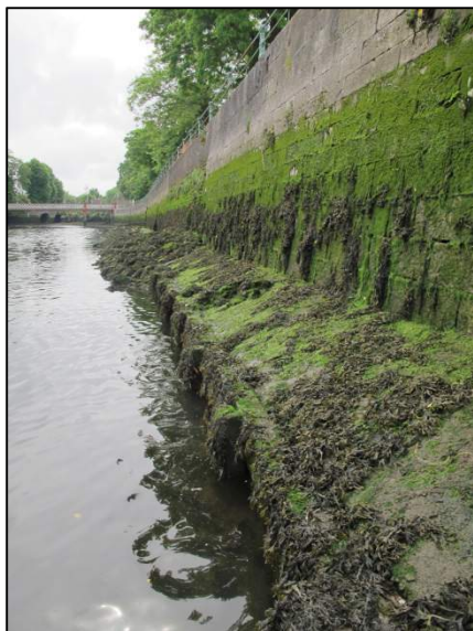
Plate 82: West-facing view along North Wall Quay showing modern consolidation of the quay's foundations.
