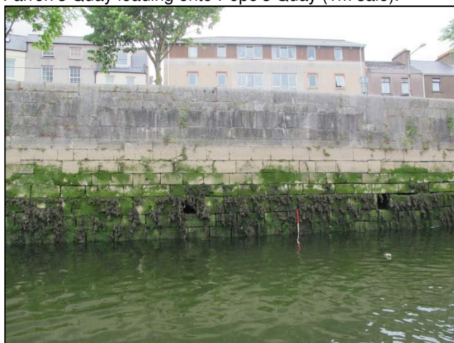
Plate 93: North-facing view showing masonry used to construct the quayside at Farren's/Pope's Quay (1m scale). Note: square profile drain features.
