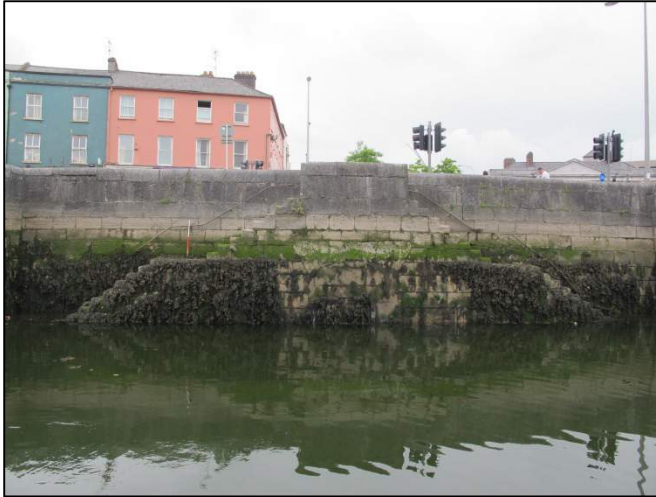
Plate 121: South-facing view of two sets of steps located a short distance downstream of Shandon Bridge (1m scale).
