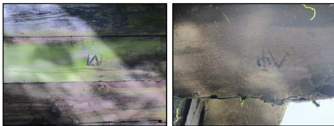
Plate 133: Detail shots of incised carpenter marks on timber used in the construction of the timber wharf.
