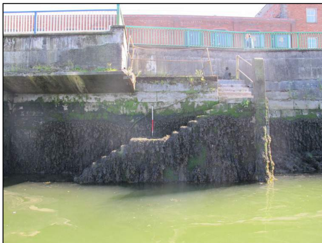
Plate 139: South-facing of first set of river access steps at Merchant's Quay (1m scale).
