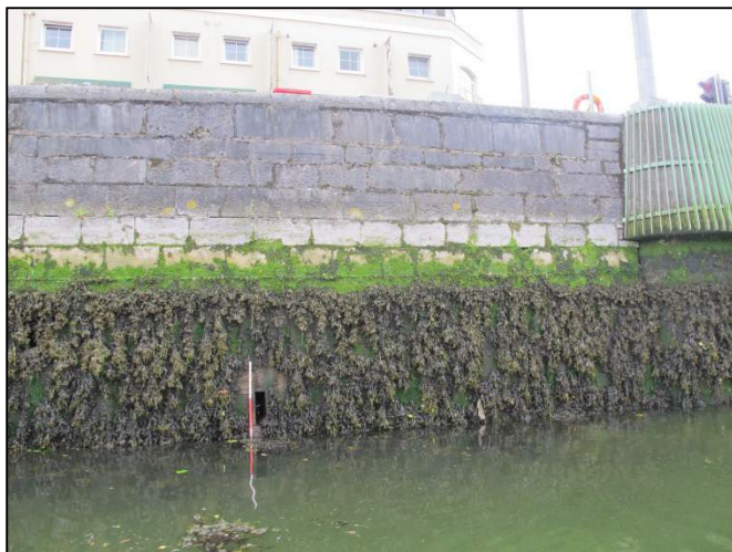
Plate 118: South-facing view of Lavitt's Quay, immediately downstream of Christy Ring Bridge Bridge (1m scale).
