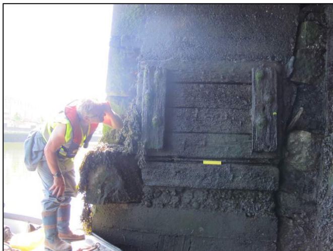
Plate 130: West-facing view of concrete and timber bracing used to consolidate St. Patricks quay at east end of timber wharf (150mm scale).
