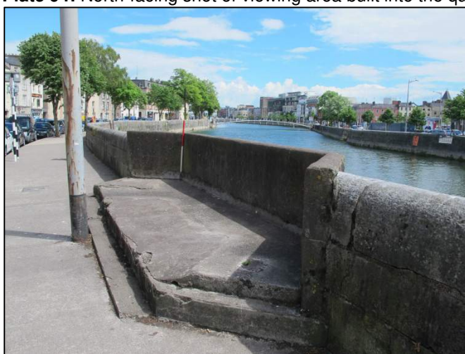
Plate 95: East-facing shot of viewing area built into the quay wall (1m scale).
