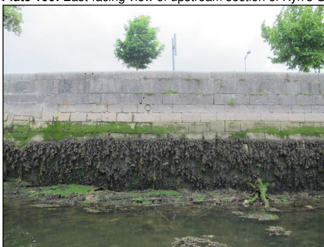
Plate 101: South-facing view of section of Kyril's Quay showing use of neat-cut limestone masonry.
