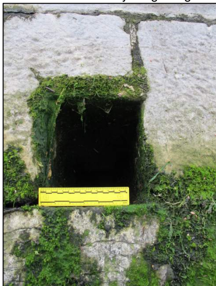
Plate 119: Example shot of drain features present along Coal Quay/Lavitt's Quay (150mm scale).
