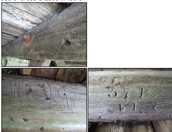
Plate 149: Example shots of incised carpenter's marks located on cross beams from the timber wharf.
