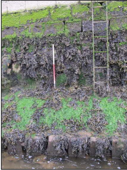
Plate 88: Detail view of timber piles and shuttering used to consolidate the quay's in-river foundations (1m scale).
