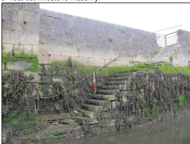
Plate 102: Southwest-facing view of upstream flight of river access steps at Kyril's Quay (1m scale).
