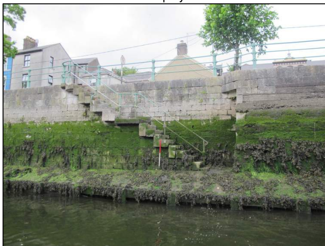
Plate 83: North-facing view of flight of masonry steps providing river access from the North Wall Quay (1m scale).
