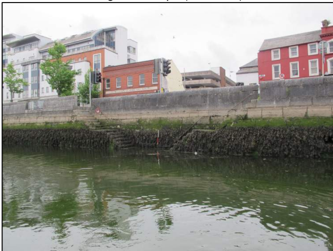
Plate 123: South-facing view of two sets of steps located 52m downstream of Shandon Bridge (1m scale).
