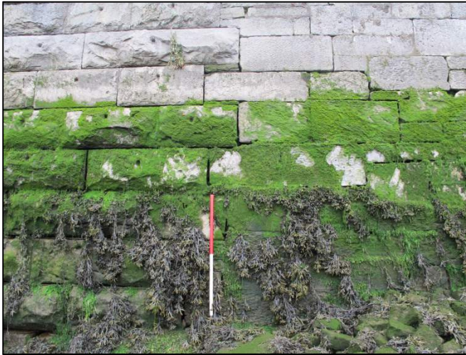
Plate 80: North-facing view showing the transition point between Wise's Quay and the con-joining North Mall Quay (1m scale).
