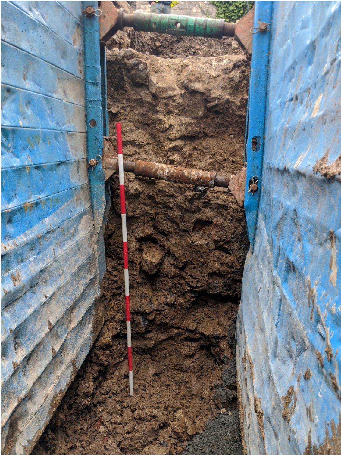
Figure 55 Northern elevation of quay wall in TT4-1.
