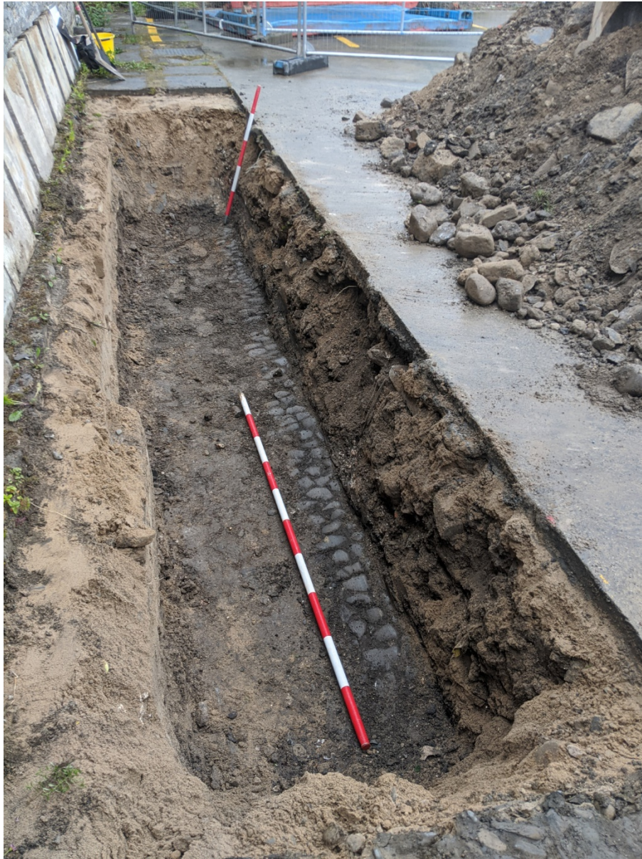
Figure 58 Looking west along TT4-2, note cobbles.
