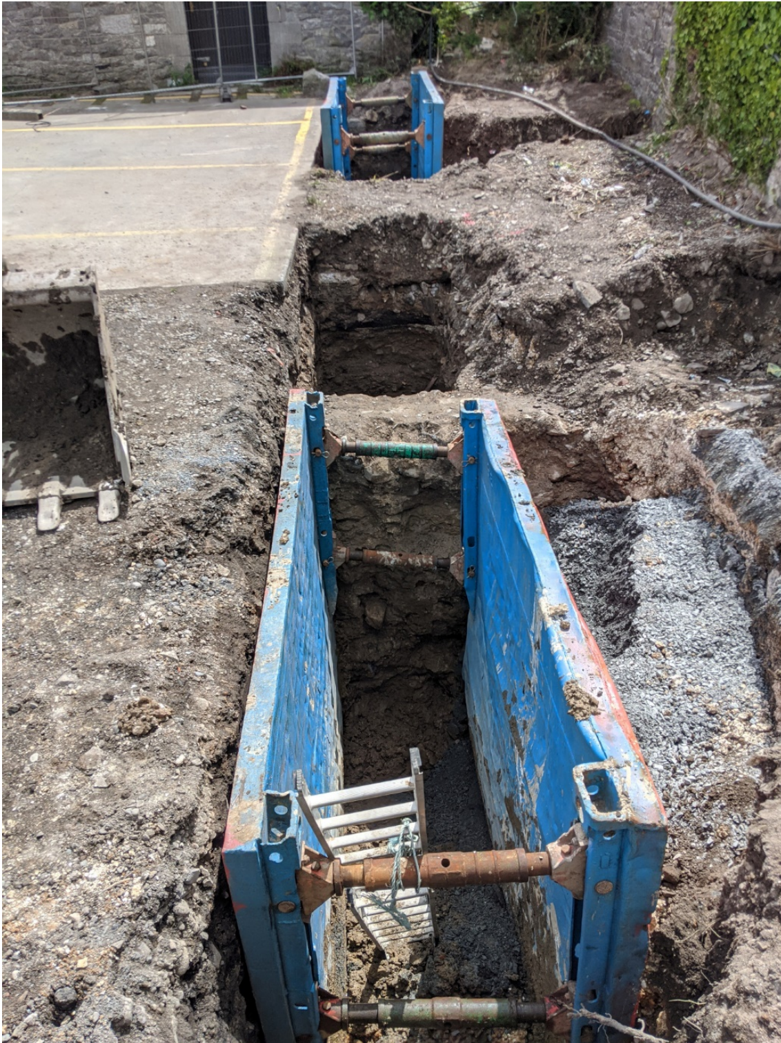
Figure 54 South-facing view of TT4-1A & B, with quay wall in middle ground.
