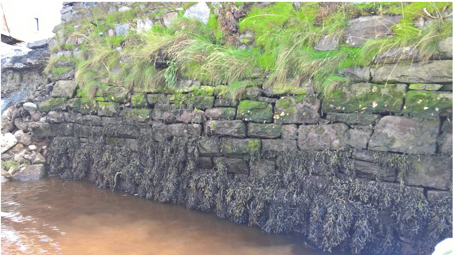
Ramelton Quay Wall
