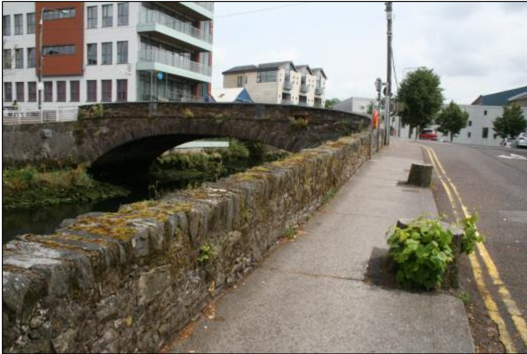
Plate 10.100: View of Wandesford Quay showing random rubble wall and Parliament Bridge from west
