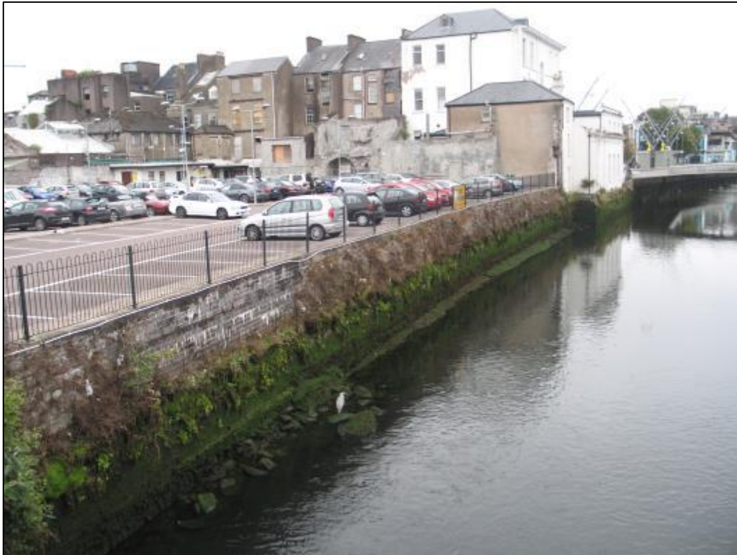
Plate 10.93: View of tarmac-covered City Car Park and modern repairs to random rubble river wall from west
