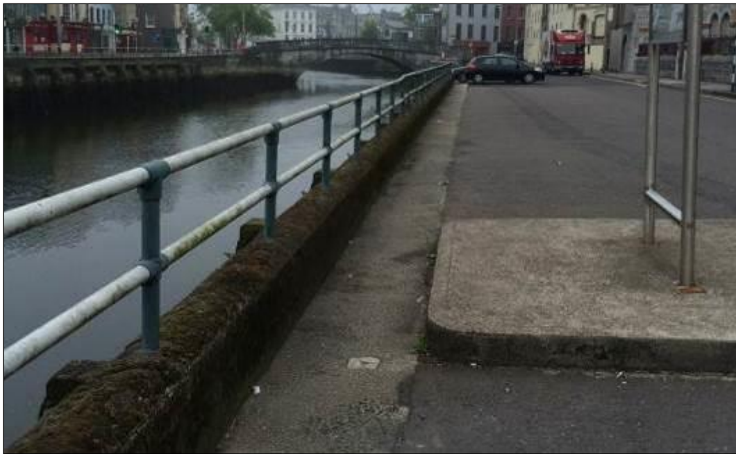
Plate 10.77: View of line of granite blocks set along top of quay walls in west end of Father Mathew Quay
