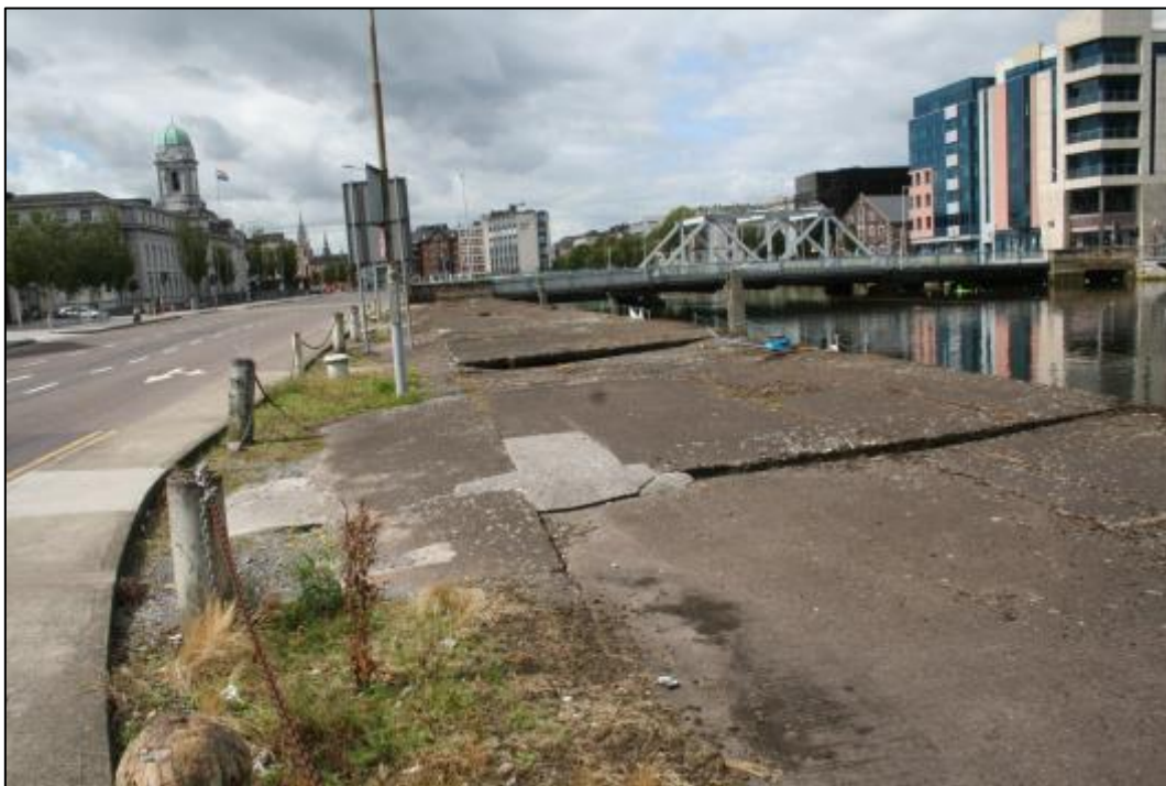
Plate 10.68 View of degraded surface of Albert Quay wharf from east (prior to recent footpath works)
