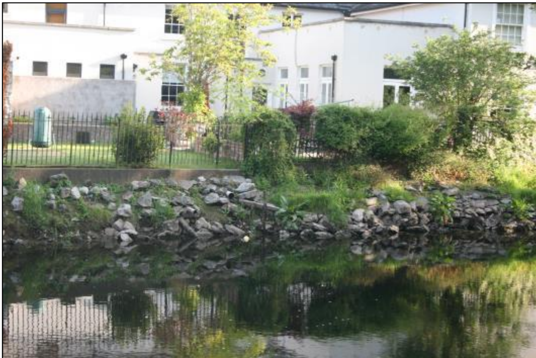
Plate 10.113: View of rubble revetment along river to rear of Western Road house west of UCC entrance
