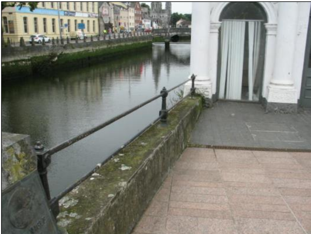
Plate 10.90: View of remnant traces of metal railing set in concrete kerb at west end of Grand Parade
