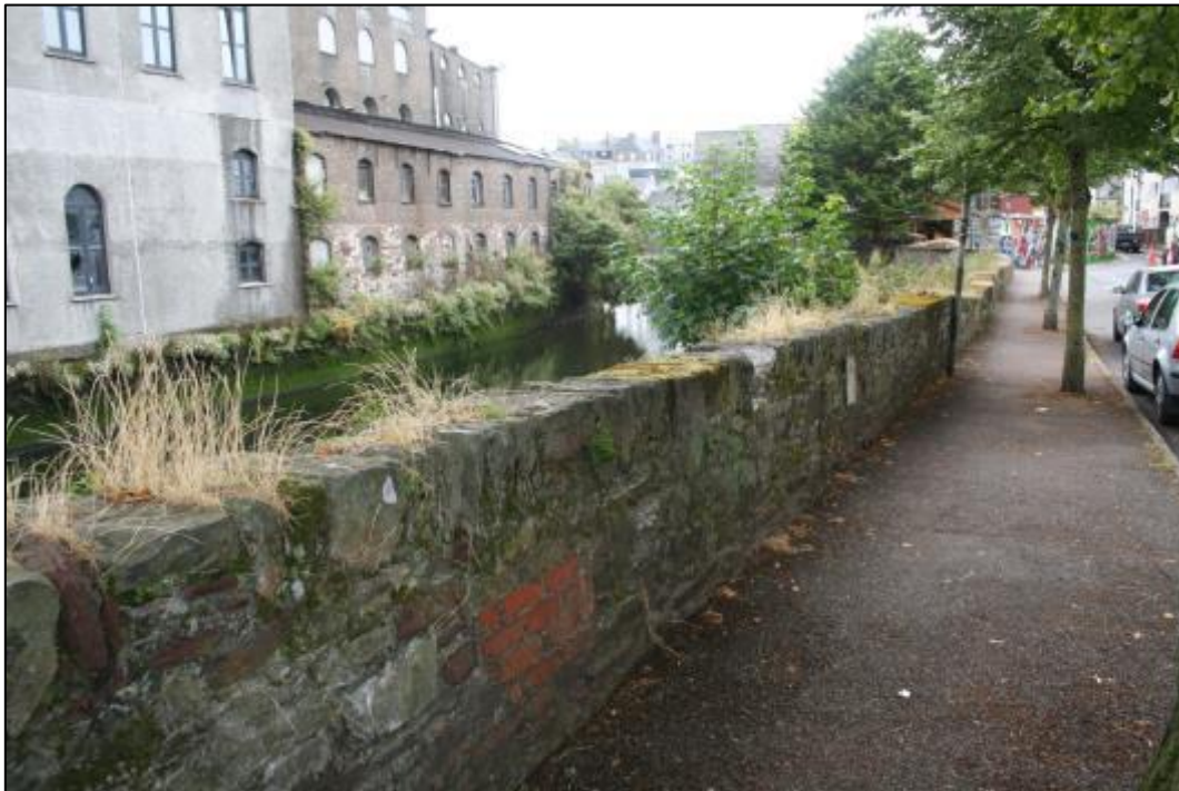
Plate 10.99: View of Crosses Green random rubble parapet wall from north
