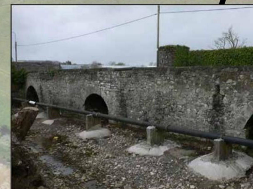
Ballinasloe East Bridge, a National Monument dating from c.1579 and possibly the longest remaining medieval bridge in Ireland. Widened in 1745 with later 19th -century span over River Suck.
