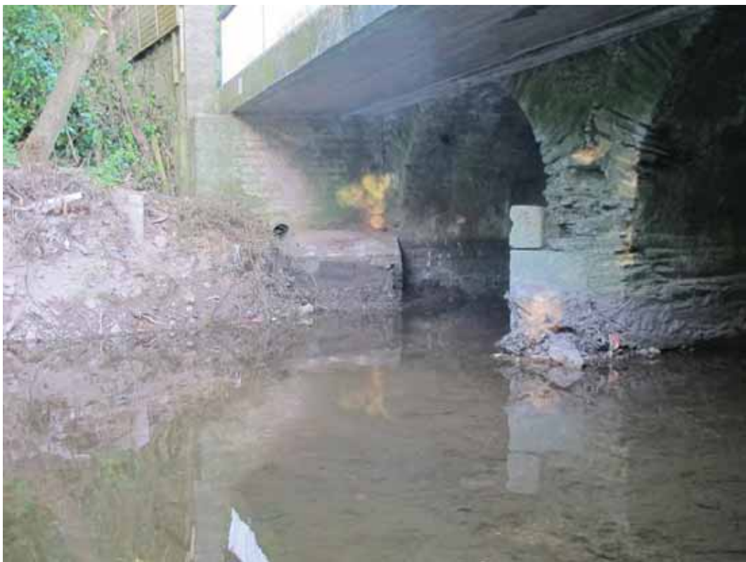
Plate 34: View of CHS 12, bridge with pedestrian bridge extension and recent earthen embankment to northeast..
