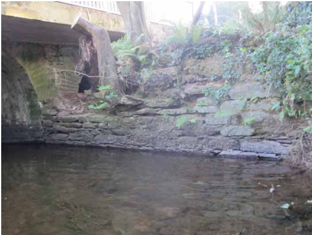
Plate 35: View of CHS 12, bridge, blocked up arch on northwest.
