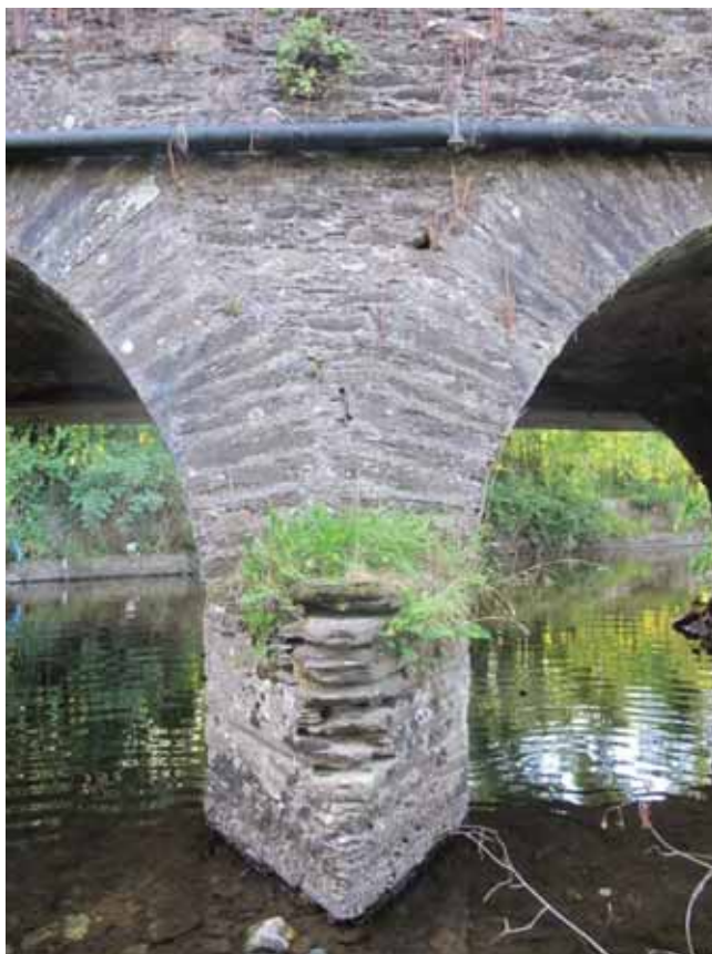
Plate 38: View of CHS 12, bridge, cutwater on downstream elevation.
