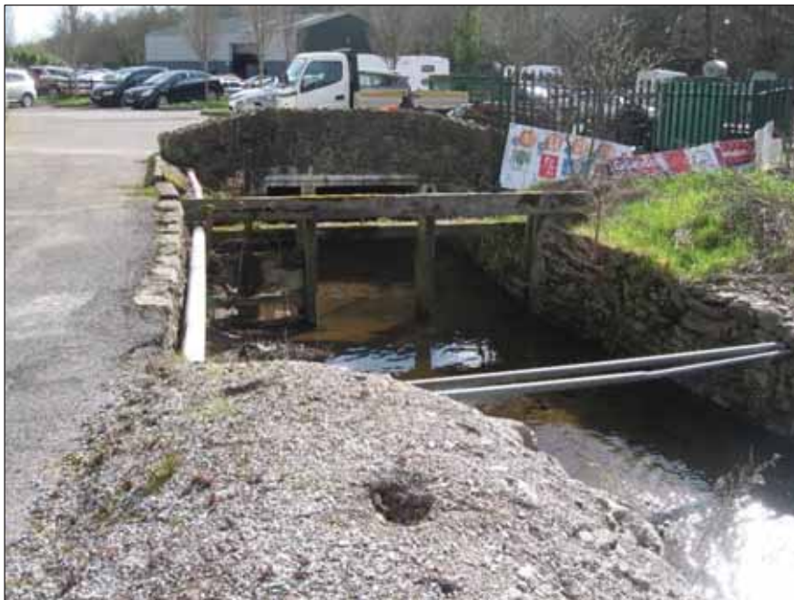
Plate 6: Mill race 3 opening in Grandon's Garage showing remains of sluice gate, before entering culvert, looking southeast
