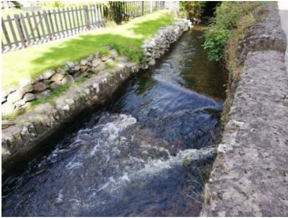
Figure 5-19. Observed small weir structure at location where Brooklodge walls are proposed (to be removed as part of the works)
