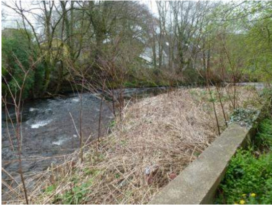
Figure 3-15 Defences downstream of the Glanmire shopping centre, adjacent to the housing estate (Point 11)
