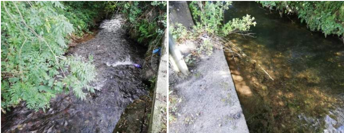
Figure 5-20. Observed downcutting at existing section of channel between Brooklodge Grove Culvert and Copper Valley Vue bridge, where bed lowering and widening is proposed
