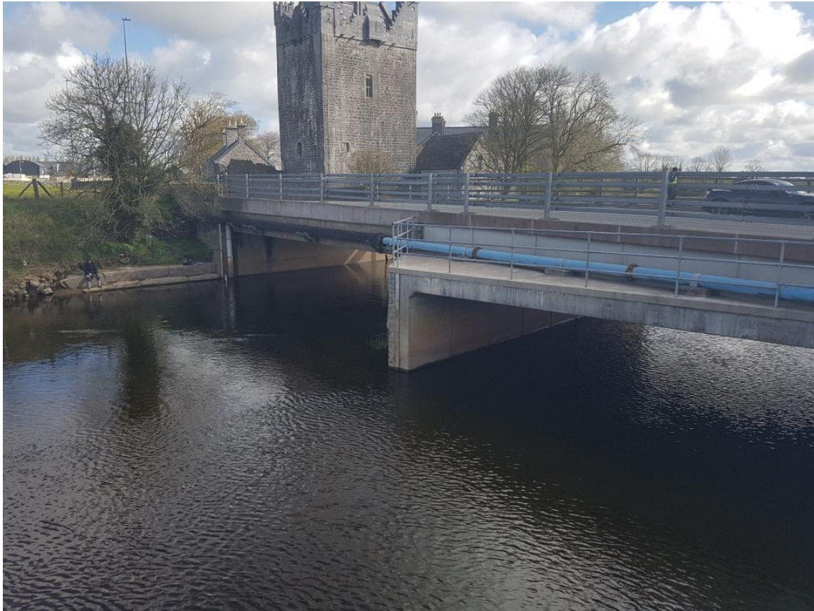
Plate 4-1 Gauging View of Downstream face of Claregalway Bridge with gauge site and stilling chamber attached to north concrete abutment and new flood eye opening in the foreground of the photo
