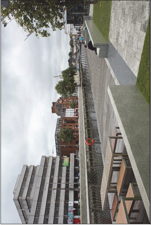
Proposed view of flood defence walls doubling as public seating with “ilt-up” or demountable flood barriers to fill gaps
