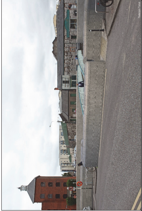
Proposed view of new flood defence walls to be closed off with flood gates when necessary
