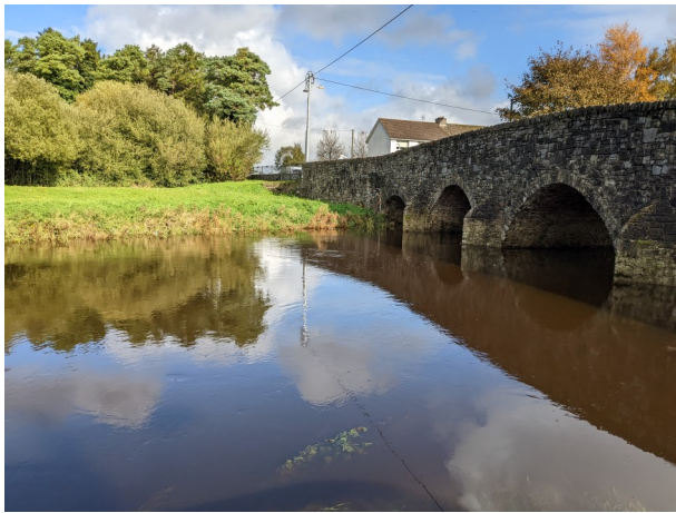
Figure 2 - Spa Street Bridge
