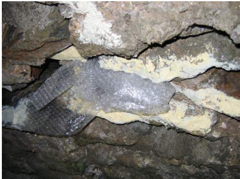
Photograph 6.10: Example of a bat-suitable crevice filled/blocked with bubble wrap to prevent bat occupancy during proposed works (Photograph courtesy of Caroline Shiel).
