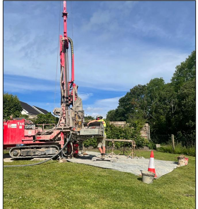
The image above shows the ground investigation contractors rotary core borehole rig set up in the near the River Finnihy in June 2024.
