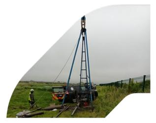
RPS are developing the specifications for the 2<sup>nd</sup> phase of the Detailed GI works. The 2<sup>nd</sup> phase of investigations will provide a detailed understanding of the ground conditions where flood defences are to be proposed.
