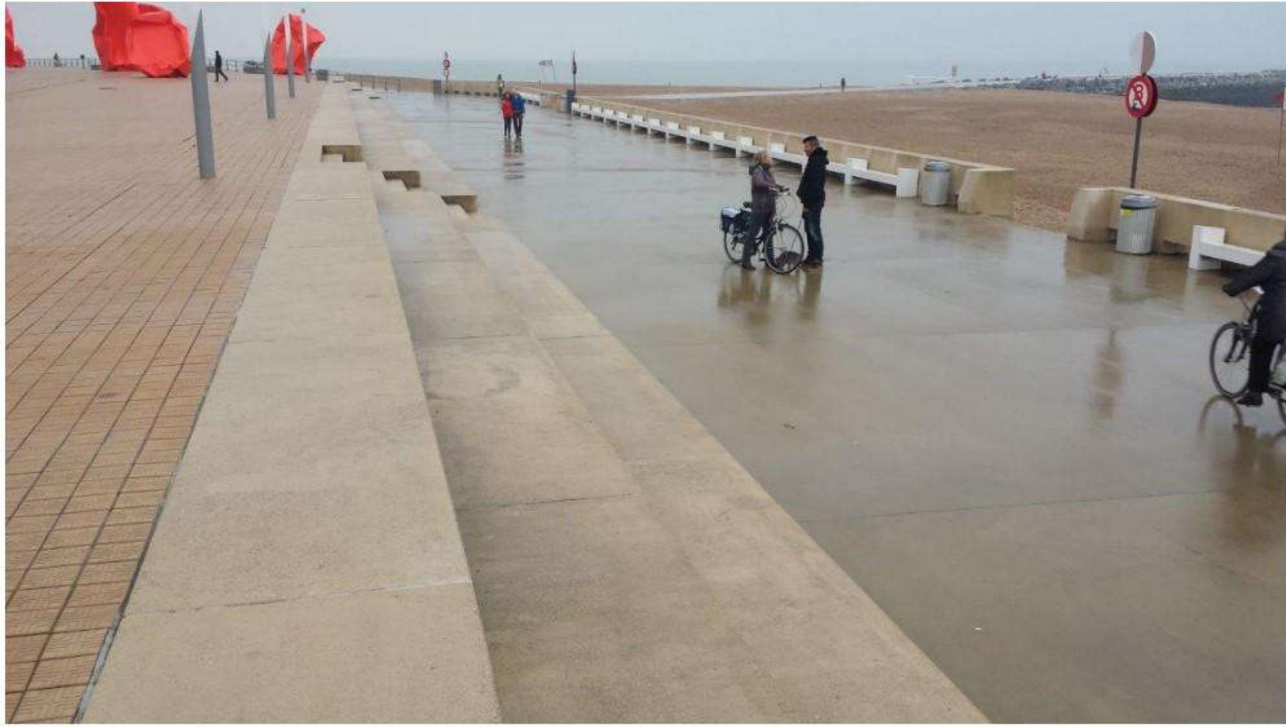
Stilling wave basin at Oostende, Belgium – designed to reduce wave energy and protect the urban waterfront during coastal storms.
