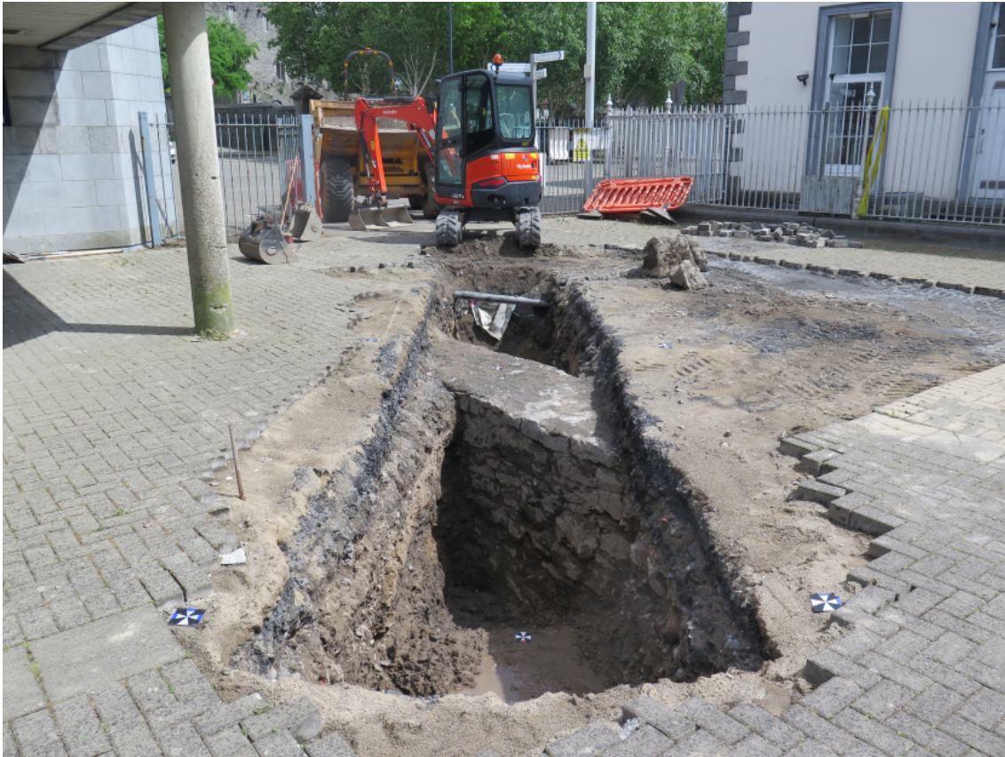
Figure 41 Looking east across TT2-1, the Old City Gaol wall built in 1811-1813.
