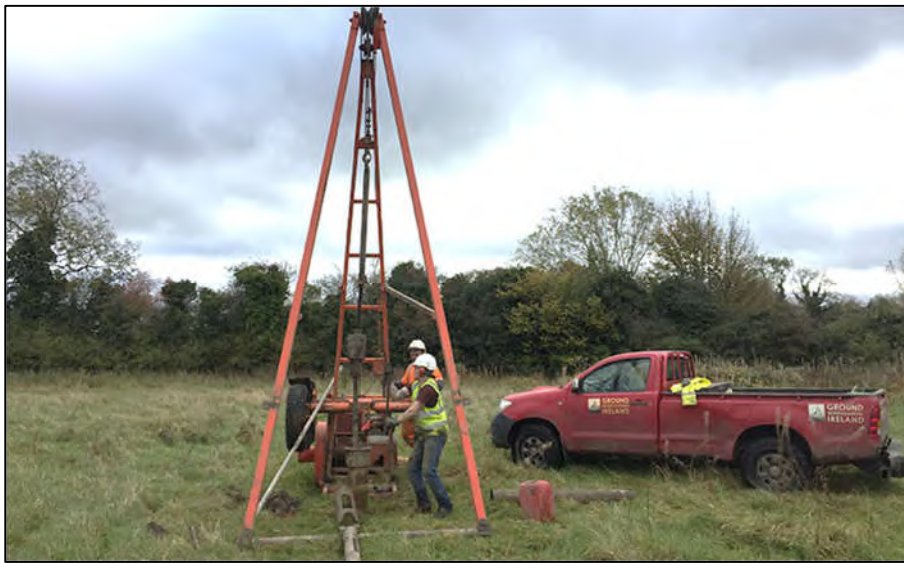
Figure 5.1. Photo of typical borehole arrangement
