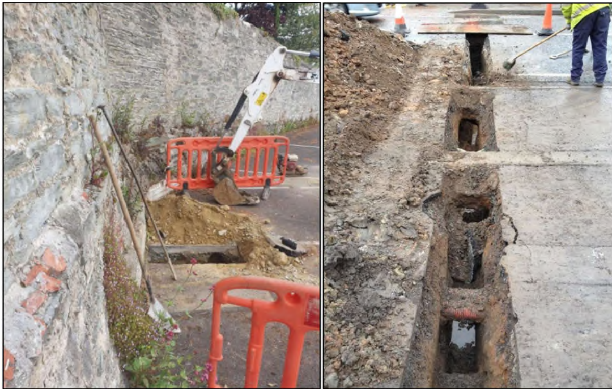
Figure 5.3. Photo of typical Inspection Pit arrangement (hand dug on the left, machine dug on the right).
