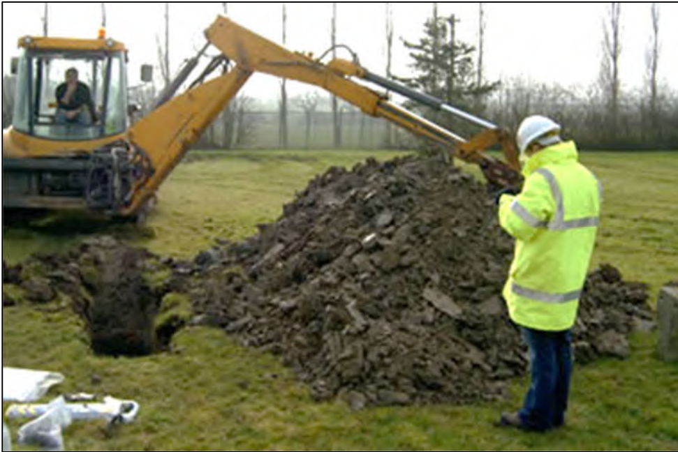
Figure 5.2. Photo of typical Trial Pit arrangement.
