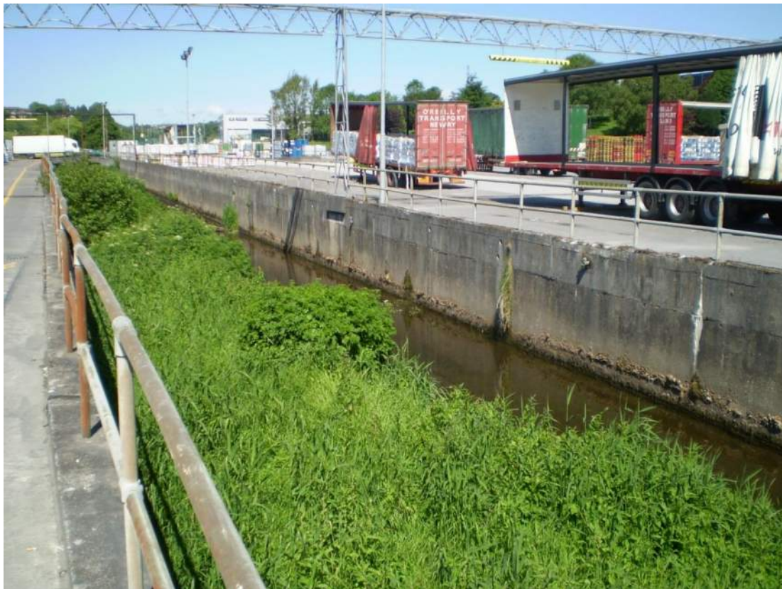
Photo of 7BRI_1184 looking upstream
