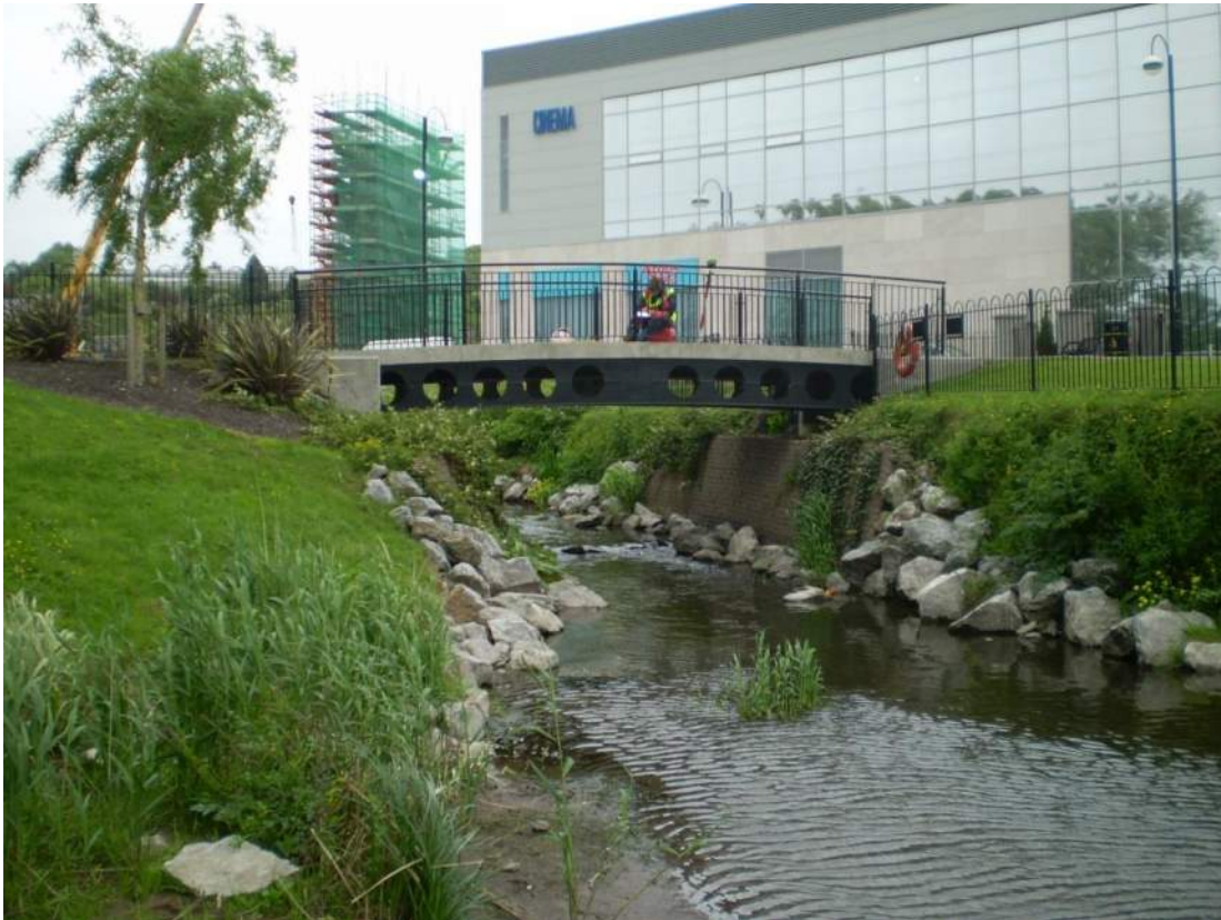
Photo of 7BRI_743 looking upstream
