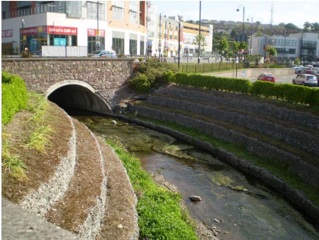
Photo of 7BRI_487 looking upstream
