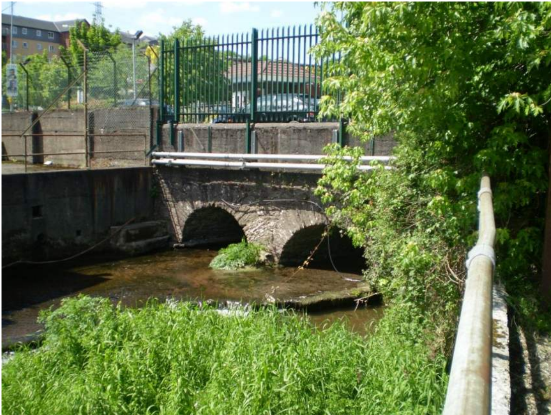
Photo of 7BRI_1406 looking upstream
