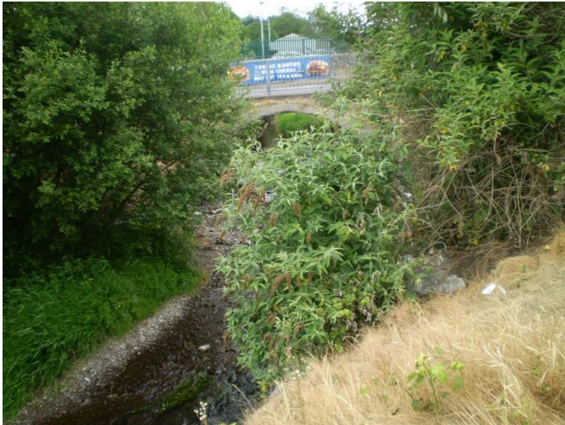
Photo of 7BRI_1432 looking upstream
