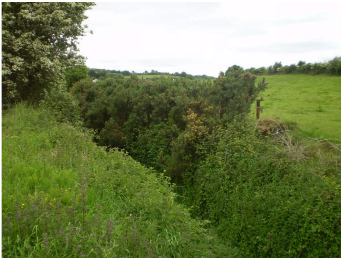
Photo of 7BRI_7782 looking upstream
