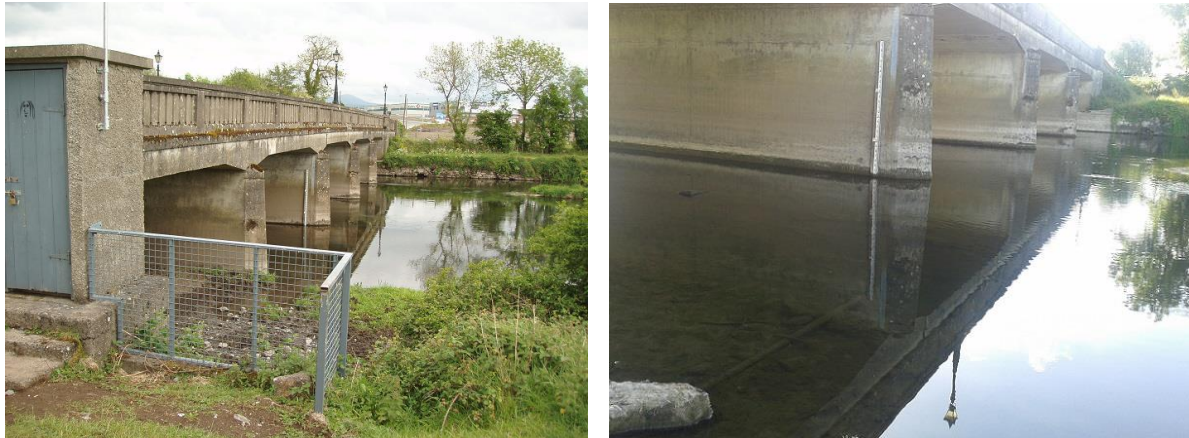
Figure 2-1: 14018 View of road bridge where station is located [left] and zoomed in view of staff gauge [right]
