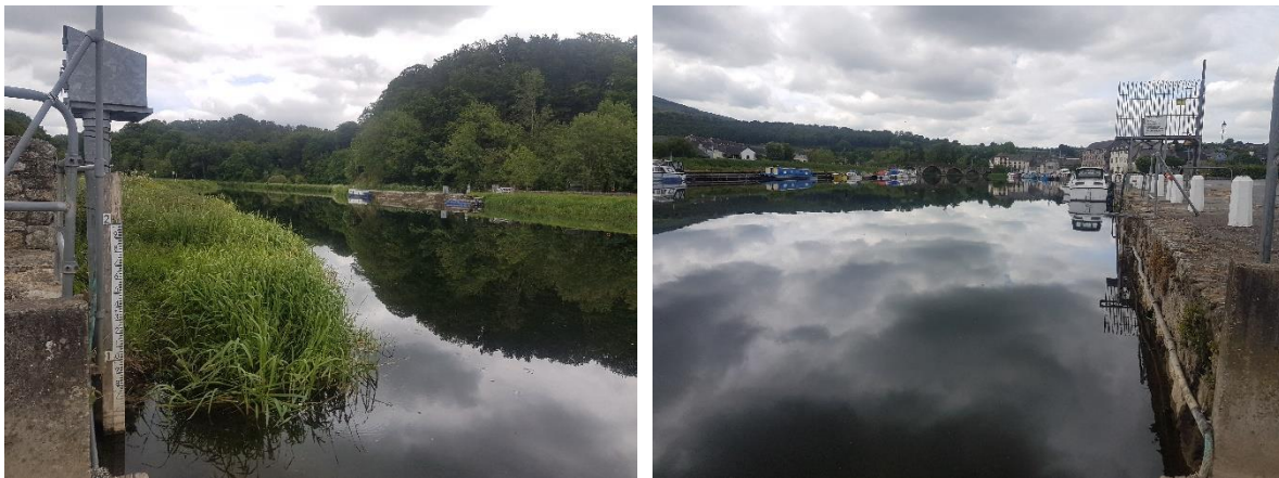
Figure 1-1: View from Graiguenamanagh u/s station upstream [left] and downstream [right]
