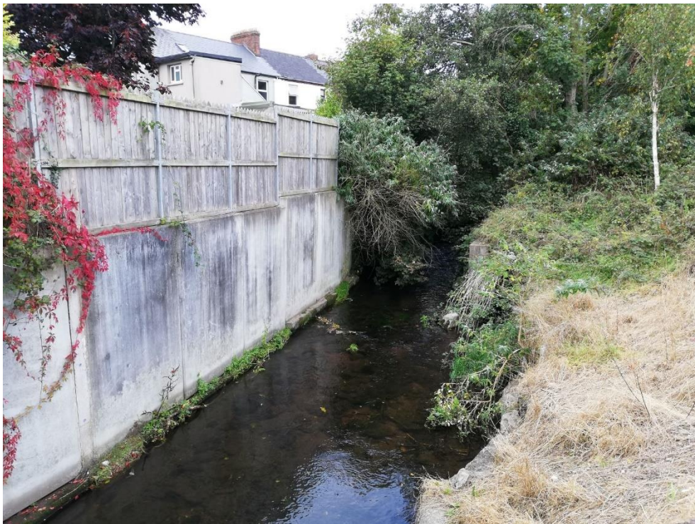
Image A2: Bride River – view upstream from within Orchard Court showing existing defences (concrete walls, boulder rip-rap).
