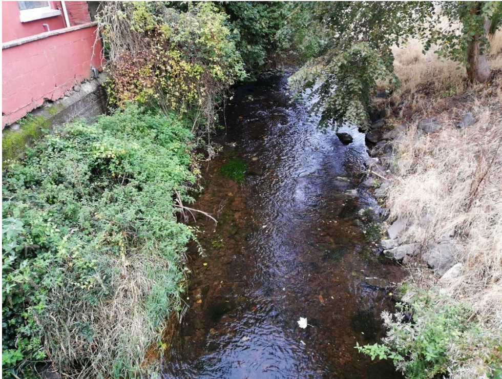
Image A1: Bride River – view upstream from entry bridge into Orchard Court showing boulder rip-rap, hard engineered walls and sprayed riparian zone. Natural in-stream substrates.
