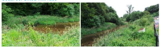
The redundant weir (noted above) feeds into the mill race shown in the photographs above. This is heavily silted due to the low velocities and limited variation in flow. Limited change is expected in this area following the construction of the new flood defences.
