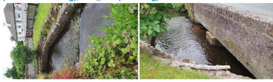
Deepening and increasing the culvert size will increase conveyance through the bridge. There will be limited impact on the channel morphology. The weir downstream of the bridge acts to trap some sediment.
