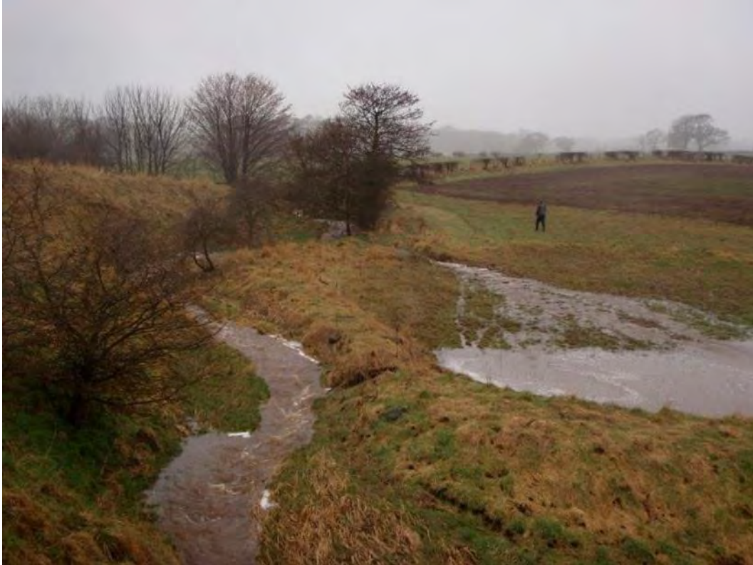
Figure 46: Offline diversion pond in Belford tapping peak flow from the river
