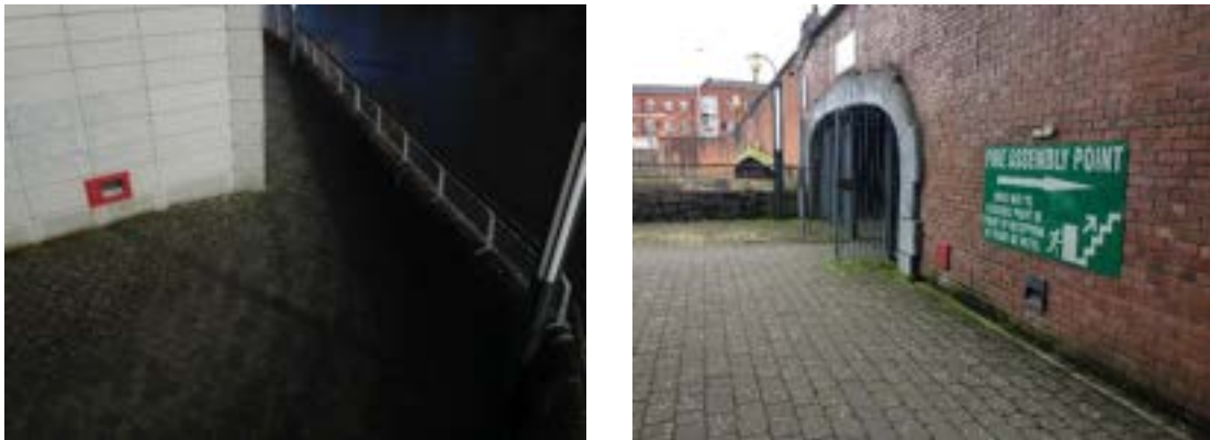
Figure 5-19: Looking from upstream from Abbey Bridge, and the underpass
