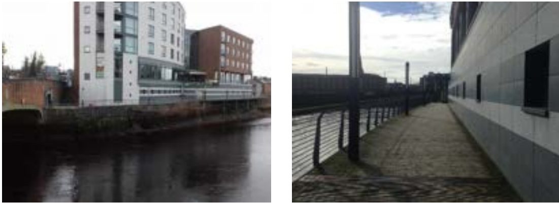
Figure 5-17: Boardwalk from opposite bank and looking downstream
