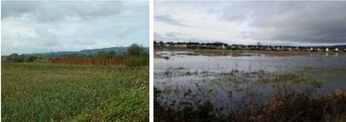
Figure 5-8: Remedial sheet piles and view across wetland
