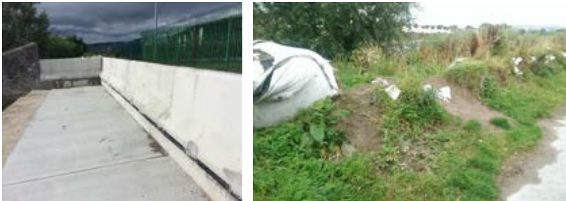
Figure 5-3: Temporary concrete barrier (left) and embankment
