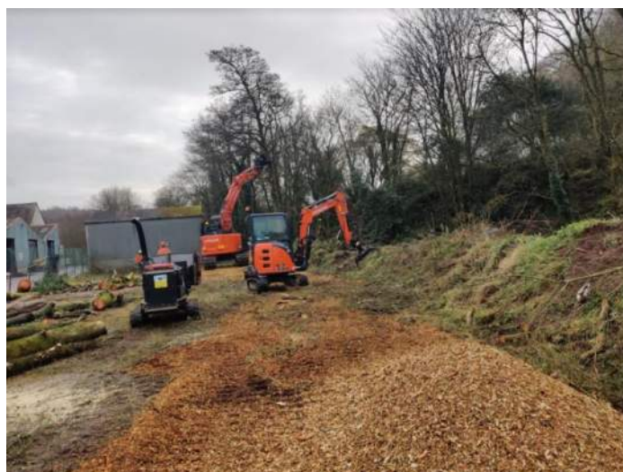
Mulching and stacking felled trees. Mulching over an area marked as Japanese Knotweed.
