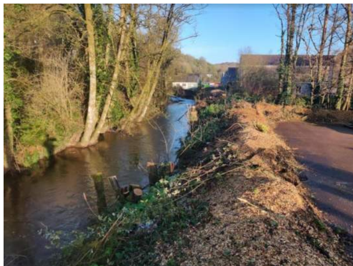
Felling completed along a riparian area. No felling into the watercourse occurred. The watercourse was protected from works activity and no pollution arising from silt or hydrocarbons occurred during works.
