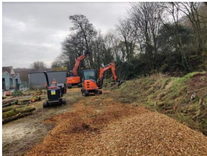
Mulching and stacking felled trees. Mulching over an area marked as Japanese Knotweed.
