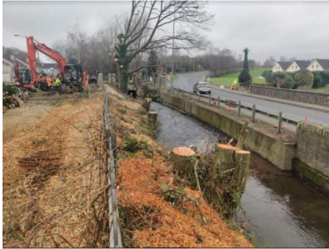
Site tree-felling and localised mulching. Felling completed and tree base and roots left in situ.
