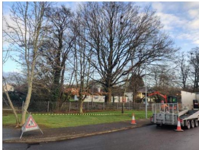
Development of a site perimeter and works area.
