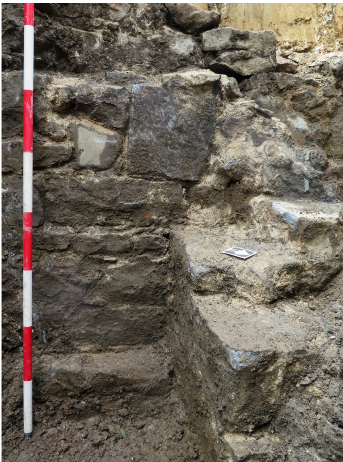
Figure 111 Junction of walls C5-5-12 and C5-5-13.
