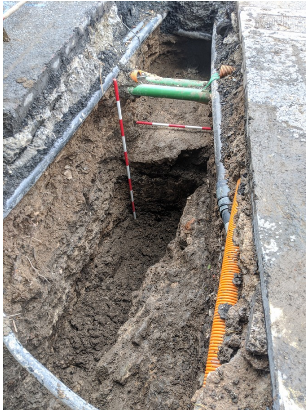
Figure 121 TT6-1 C facing northeast, showing wall and foundations
