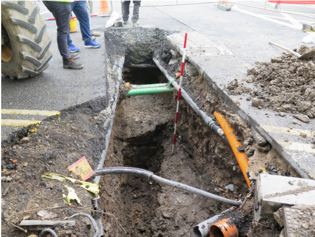
Figure 120 TT6-1 C, facing north at work in progress, exposing foundations and intersecting wall
