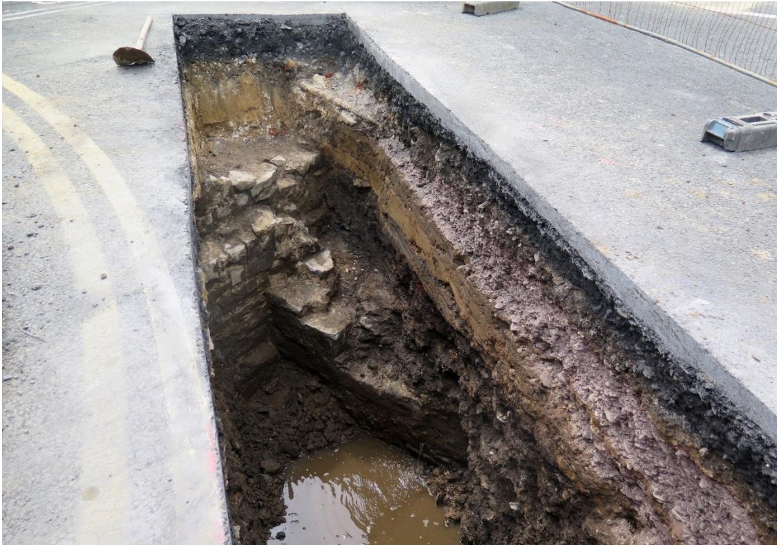
Figure 109 Water inundating TT5-5 after excavation of sounding
