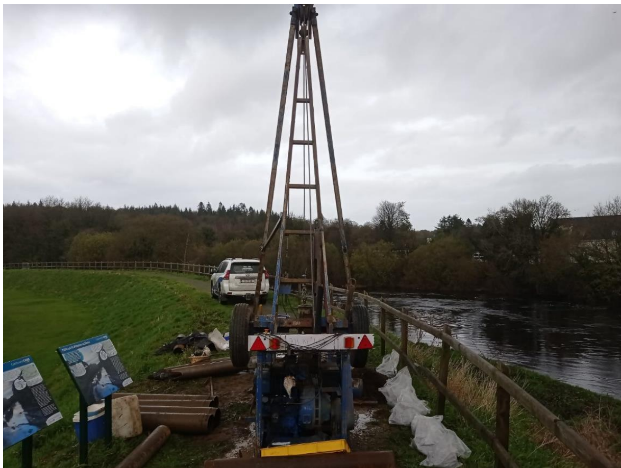
Cable Percussion Drilling along Ballybofey embankment
