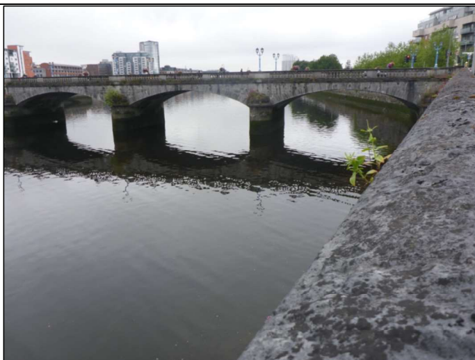
Photograph 4.1 Sarsfield Bridge and River Shannon (view to SW from N bank)
