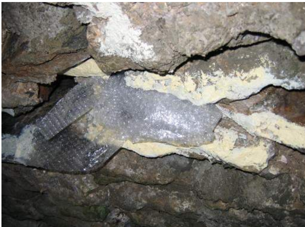
Photo 6.10: Example of a bat-suitable crevice filled/blocked with bubble wrap to prevent bat occupancy during proposed works (Photograph courtesy of Caroline Shiel).
