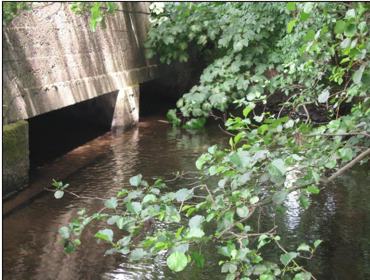
Plate 8: Western culvert openings, south-facing elevation
