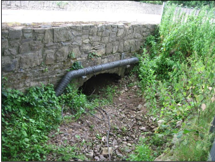
Plate 7: Eastern culvert opening, showing dry south-facing elevation
