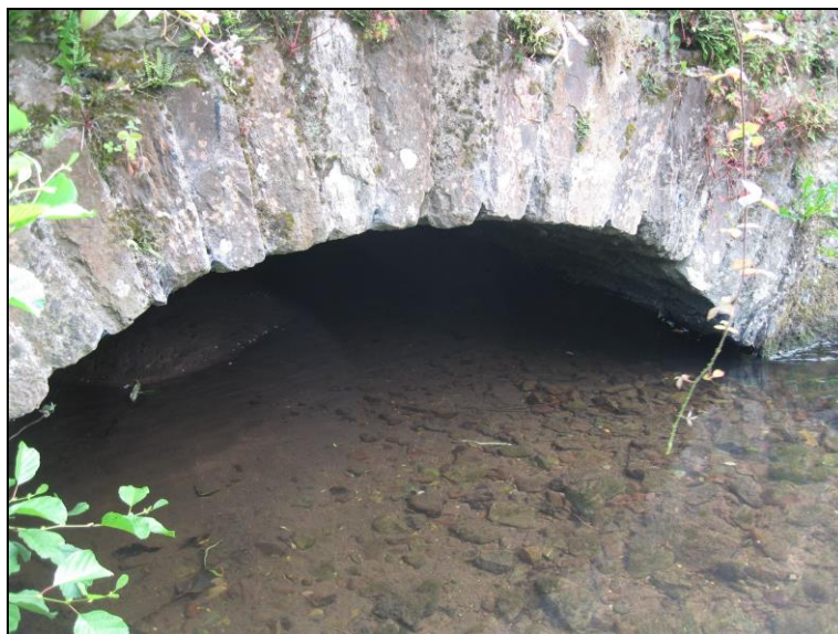
Plate 6: Eastern culvert opening, north-facing elevation
