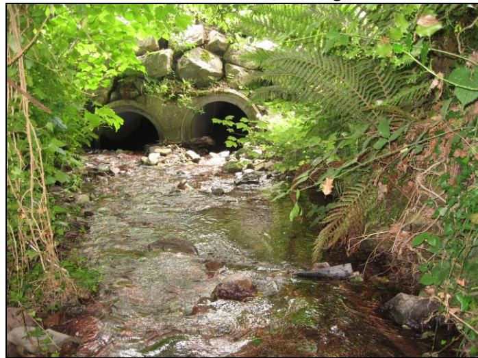
Plate 2: Bleach Hill Stream, opening of culvert under road, looking southwest
