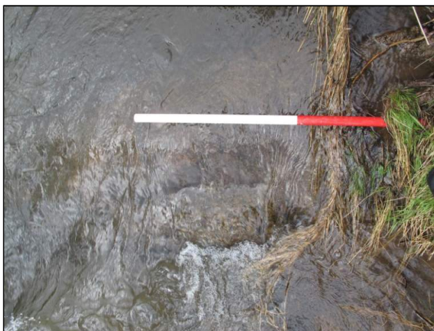
Plate 66: Concrete encased pipe that extends across the river channel (1m scale); see Figure 14 for location.
