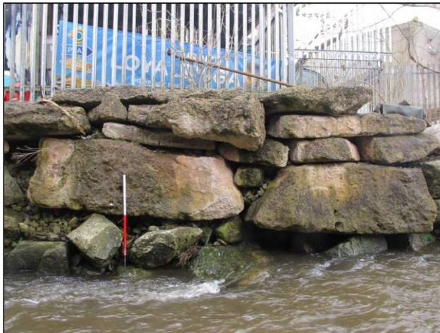
Plate 65: Rock-armour placed to protect the adjacent filling station (1m scale).
