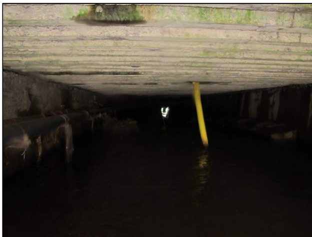
Plate 87: View from inside the culvert showing box-section concrete used in its construction.
