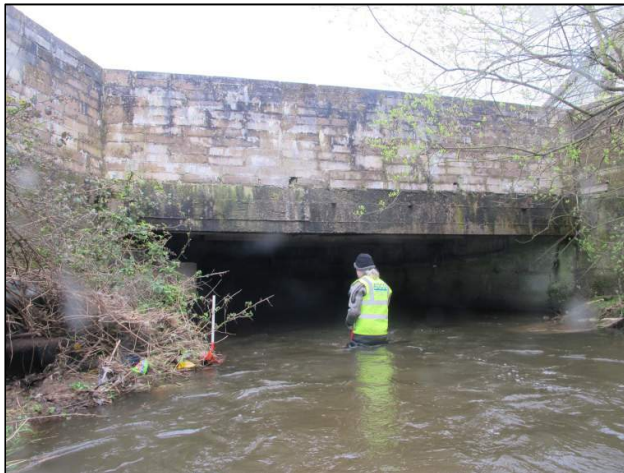
Plate 86: Upstream side of 70m long concrete culvert which accommodates river-flow past the sunbeam Industrial Estate (1m scale).
