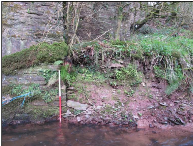
Plate 5: Exposed section of bank structure located on north side of river, located on upstream side of Kilnap Bridge (1m scale).
