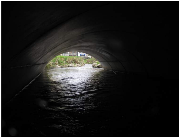
Plate 89: Internal shot from 9m-long section of modern culvert that provides access to the Sunbeam Industrial Estate.
