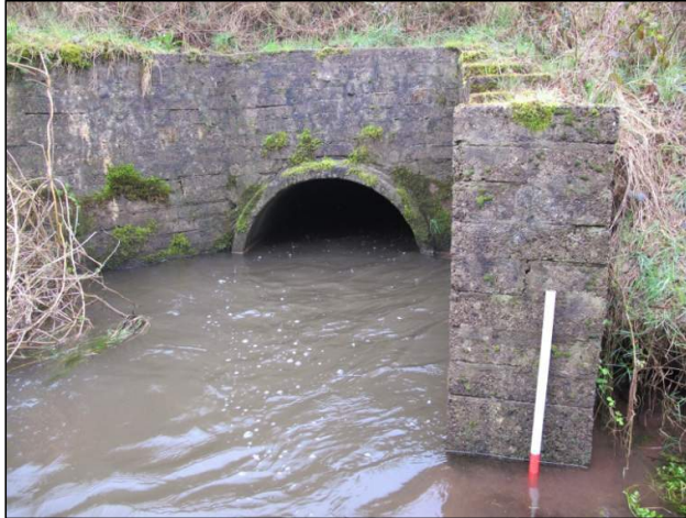
Plate 40: Concrete Culvert and deflector located halfway along visible extent of Rathpeacon Stream (1m scale).
