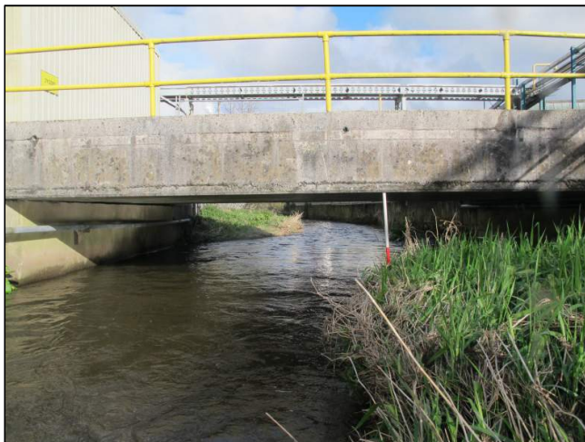
Plate 75: Modern bridge culvert providing vehicular access between factory units (second of two such culverts).
