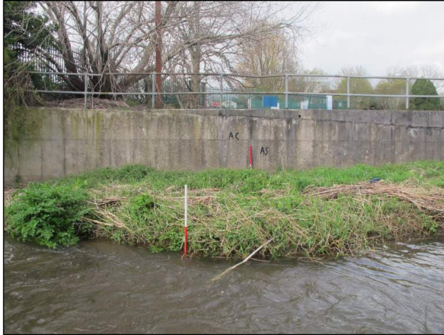
Plate 73: North-facing view of River Bride showing the height of the concrete retaining walls that delineate the channel as it flows through the Dulux Factory site (1m scale).
