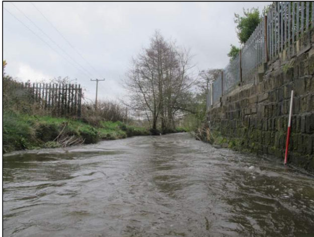
Plate 59: Modern river-walling delineating south side of the river, placed to protect adjacent dwellings (1m scale).
