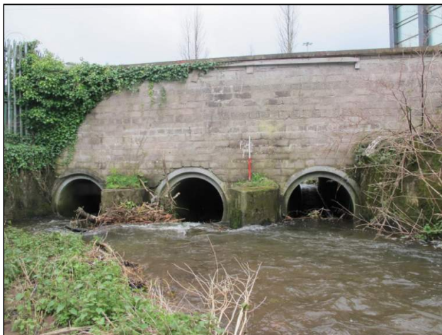
Plate 36: Upstream façade of modern culvert providing access to the North Point Business Park (1m scale).
