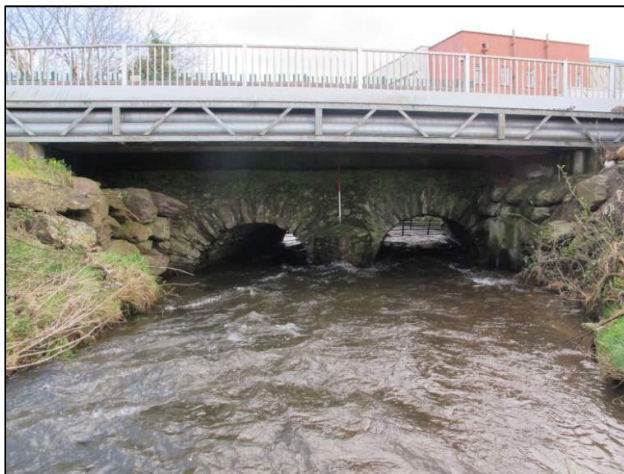
Plate 69: Upstream view of Masonry Bridge, Feature F09, which accommodates Fitz's Boreen (1m scale); see Figure 14 for location.
