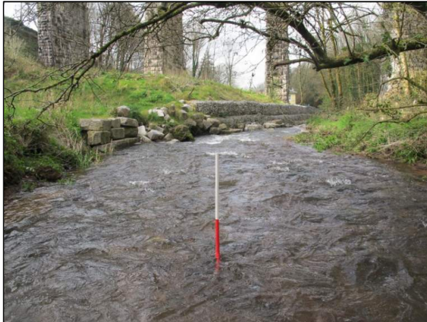
Plate 8: Southwest-view of the river between Kilnap Bridge and Kilnap Viaduct, note use of rock armour on south side of channel (1m scale).
