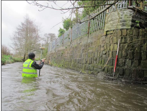
Plate 58: Modern river-walling delineating south side of the river, placed to protect adjacent dwellings (1m scale).
