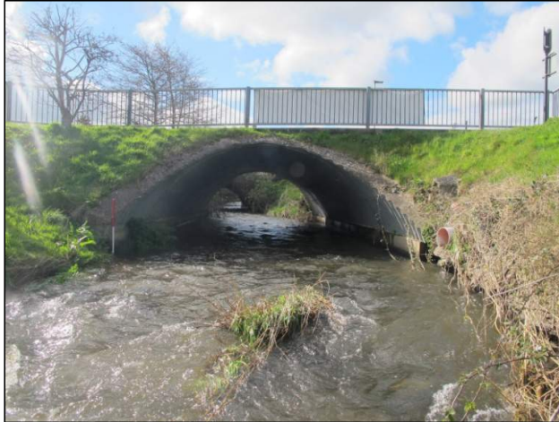
Plate 70: Downstream side of concrete culvert placed to accommodate access to McDonald's Restaurant (1m scale).
