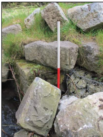
Plate 9: Rock armour incorporating masonry from Kilnap Viaduct (1m scale).
