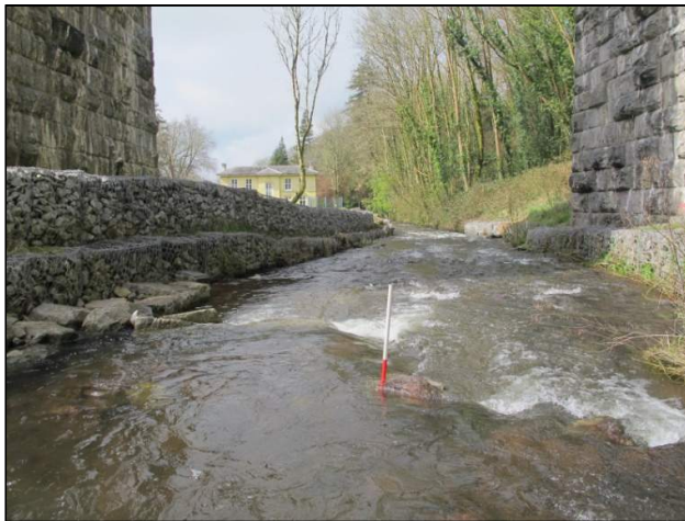
Plate 11: Southwest-facing view of river channel beneath of Kilnap Viaduct, note use of delineated by stone-filled gabions (1m scale).
