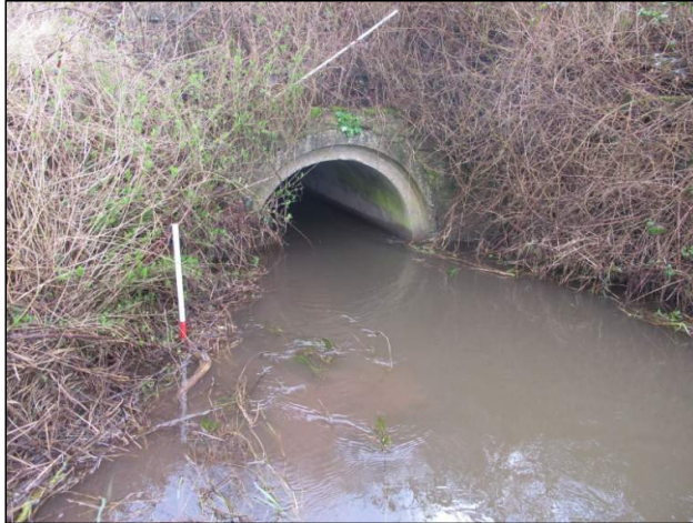
Plate 43: Concrete culvert that channels river-flow beneath the N20 roadway and associated slip-roads (1m scale).
