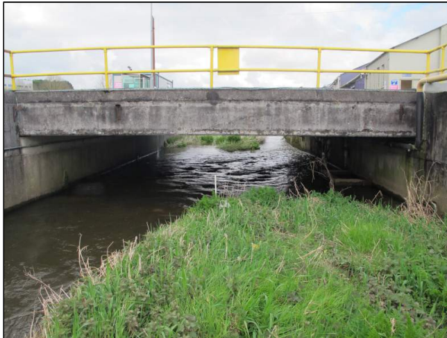
Plate 74: Modern bridge culvert providing vehicular access between factory units (first of two such culverts)
