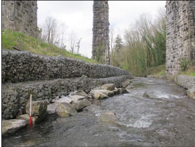
Plate 10: Southwest-facing view of river channel immediately upstream of Kilnap Viaduct, note channel delineated by stone-filled gabions (1m scale).
