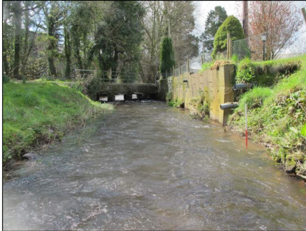
Plate 28: River channel on upstream of Feature F07, note concrete retaining wall on west side of channel (1m scale).
