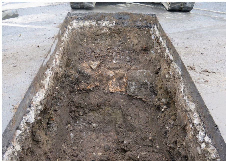
Figure 62 Wall foundations at northeast of TT6-4 (C6-4-06)
