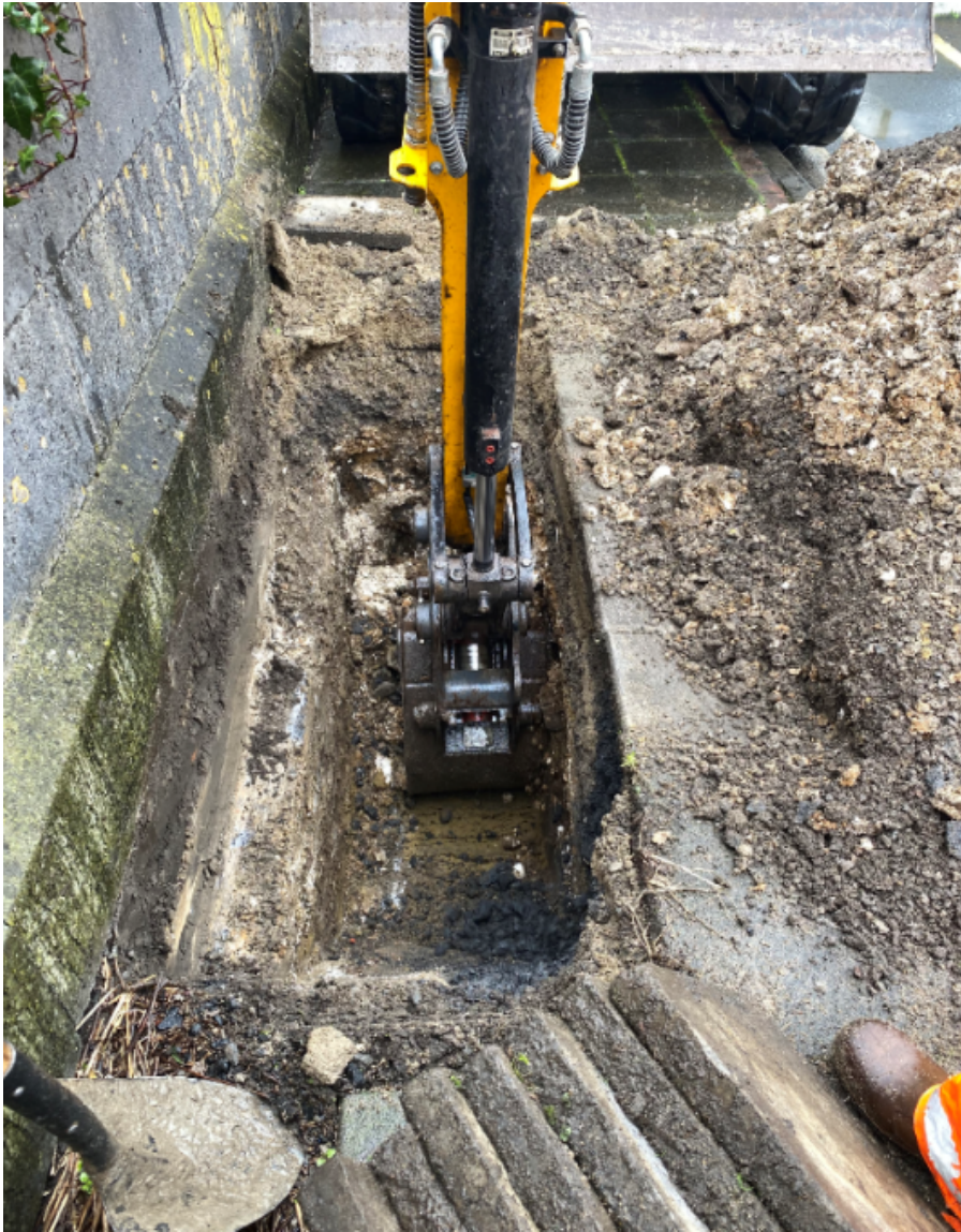
Figure 69 Work in progress FIP 309
