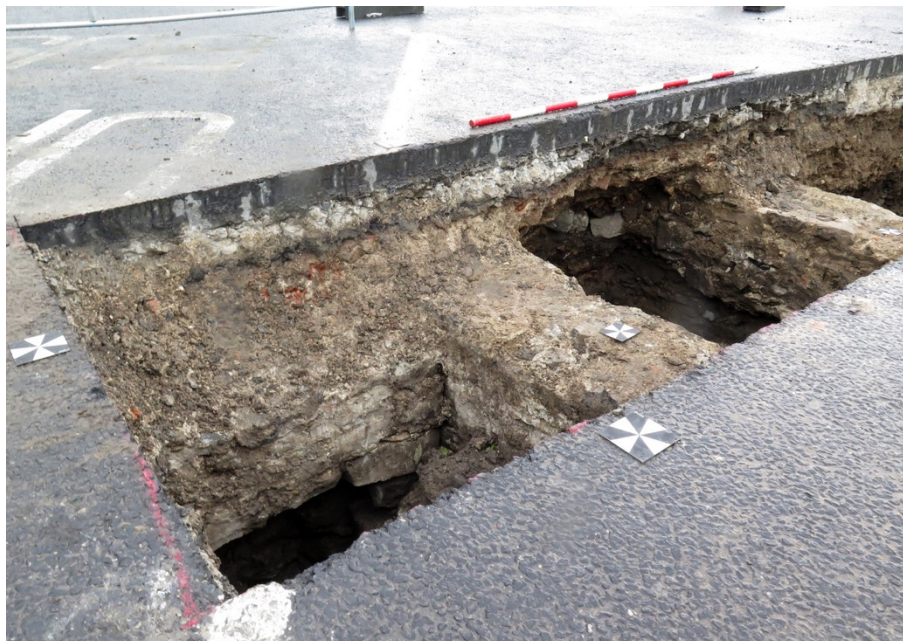
Figure 58 Wall crossing TT6-3 (C6-3-08)
