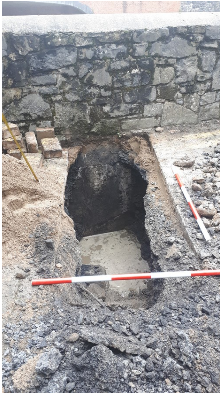
Figure 66 Quay wall FIP 303 Sir Harrys Mall
