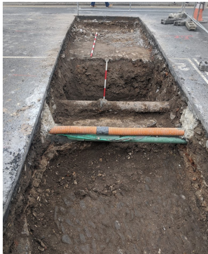
Figure 57 Stone foundation under pipe infrastructure in TT6-2 (C6-2-12), note both levels of cobbles
